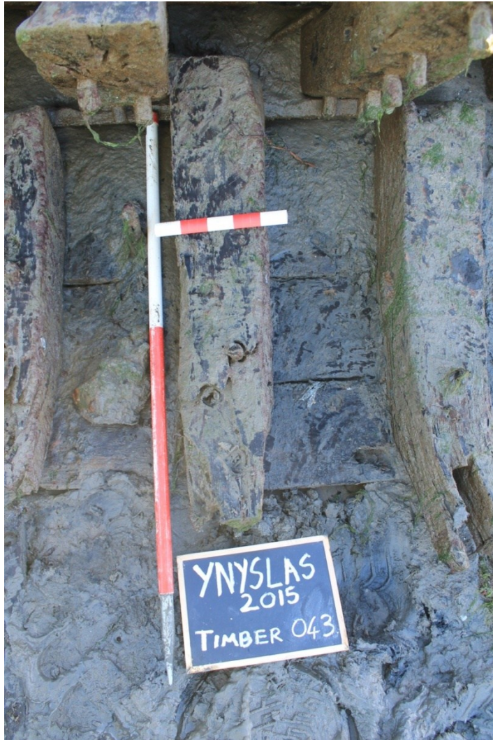
Photo 21: Fallen 1 st futtock attached to collapsed outer planking in June 2015
