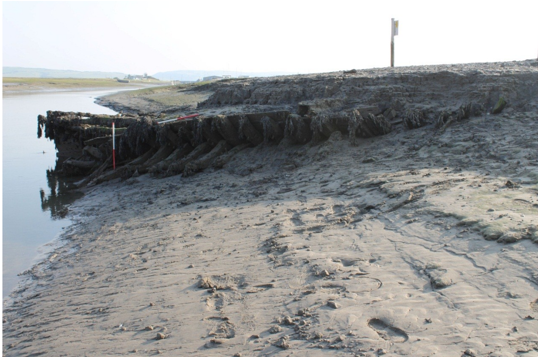
Photo 1: Showing the hulk eroding into the Afon Leri, viewing south
