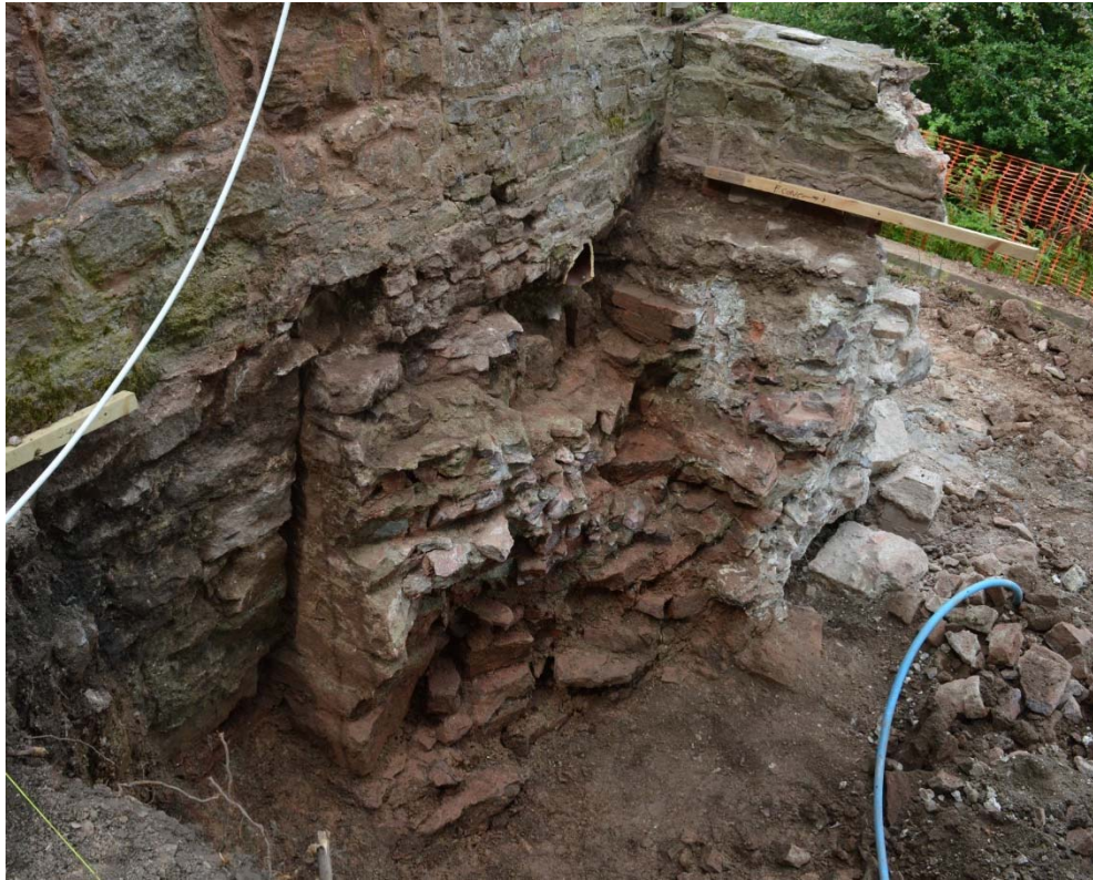
Fig. 10 The medieval curtain wall, showing the butt-joint with the 18 th -century kitchen wing
