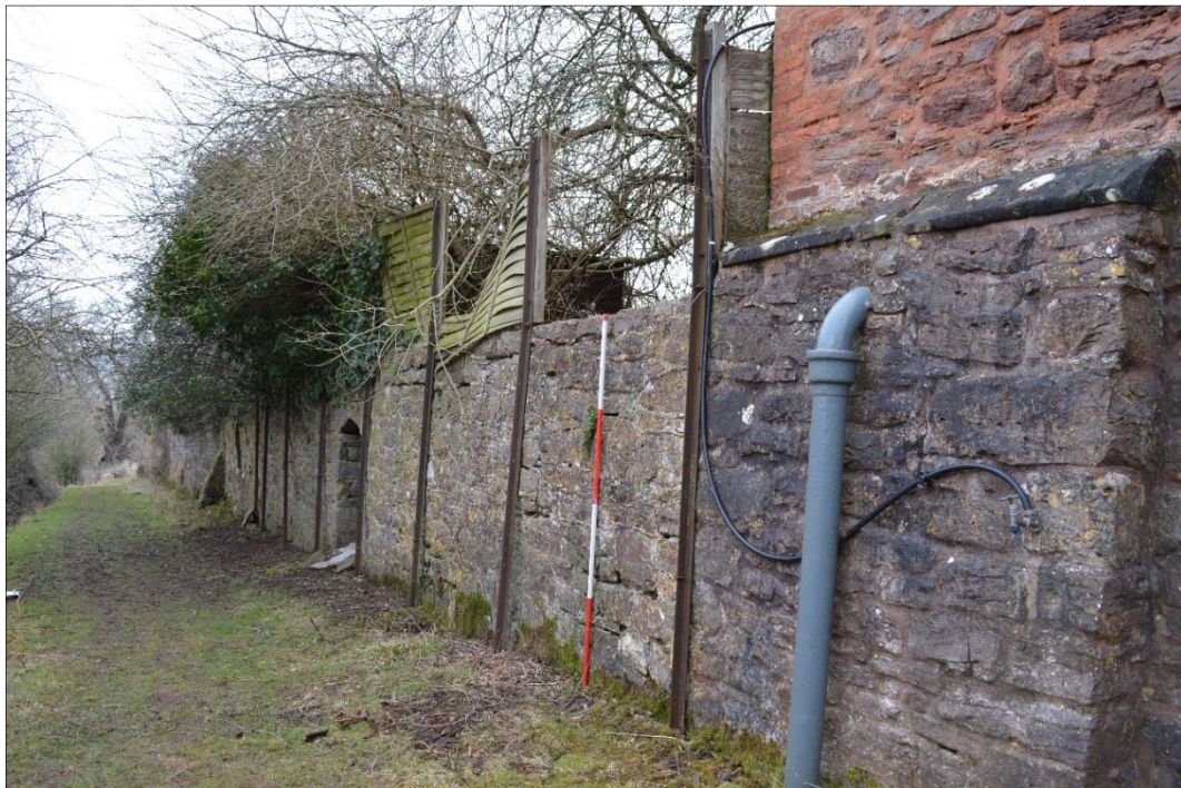
Fig. 3 The section of retaining wall recorded during the building survey.
