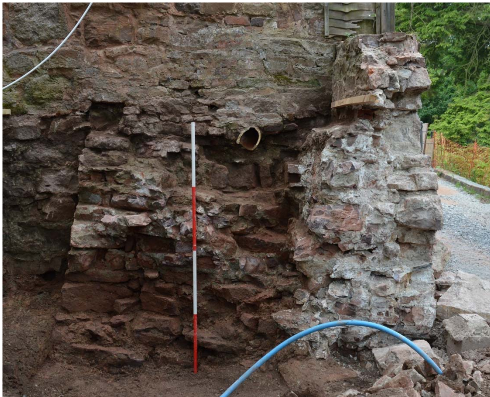
Fig. 9 North-east facing section through the medieval curtain wall
