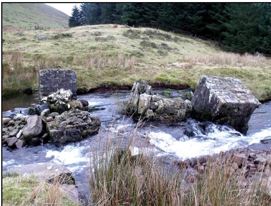
Photo 73. Showing collapse of some of the anti tank blocks of BR337F
