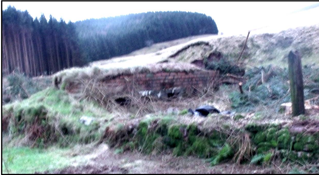
Photo 67. Facing northeast showing Pillbox BR337C and recent felling activity all round the site
