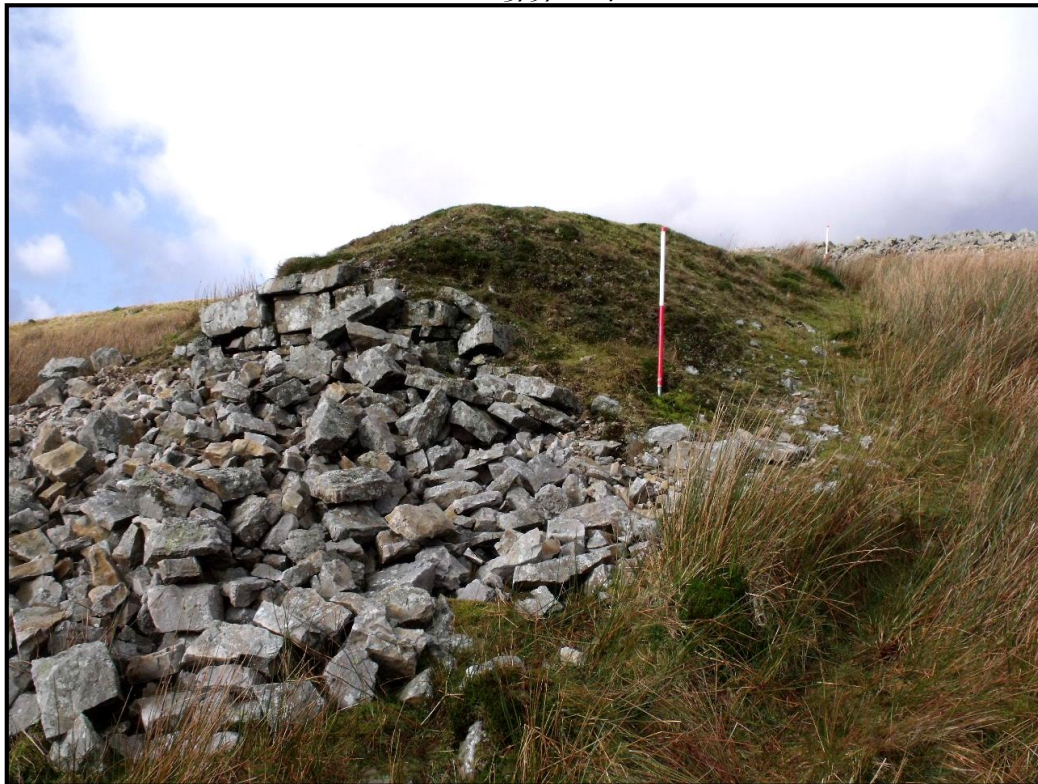
Photo 55. Facing northwest showing collapsed structure at side of tramroad of BR237 (PRN 114089)
