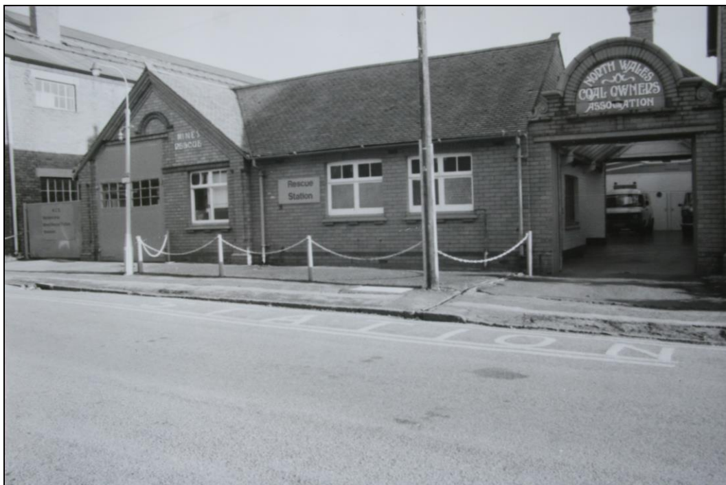
Frontage before infilling of main entrance
