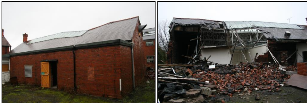
Gallery extensions to south and north sides of drill hall
