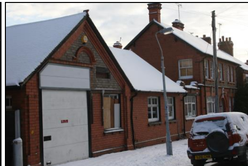
Frontage looking from north
