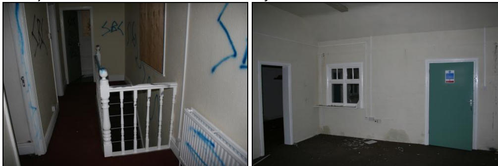
Staircase and landing to house
