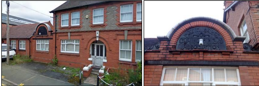
Frontage showing gable with inscription prior to removal
