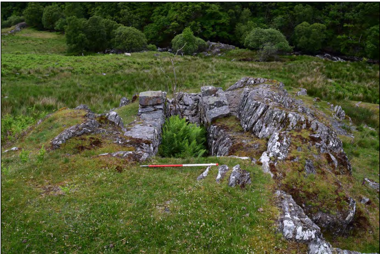
Plate 72: The lower wheel pit at the Nant y Car mine (ID number 524). Looking north-northeast.
