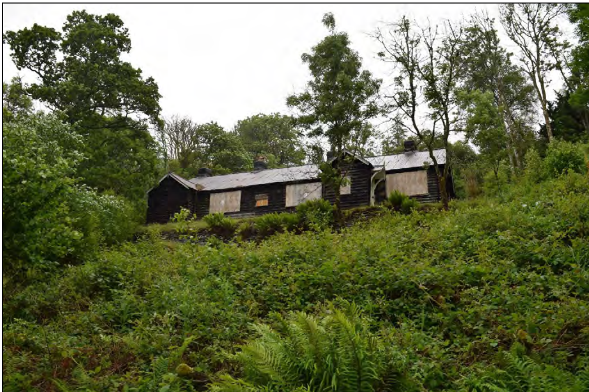
Plate 53: The Engineers House (ID number 1222) is the last of the late 19 th century Dam Builders houses and offices standing in its original position. Looking north.
