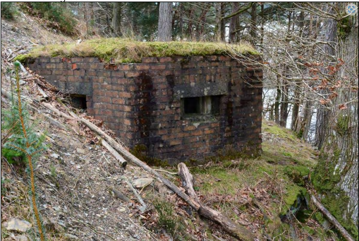
Plate 96: Pillbox ID number 399, one of the three surviving Second World War pillboxes which protected Garreg Ddu dam. Looking south. (Photo © David James).
