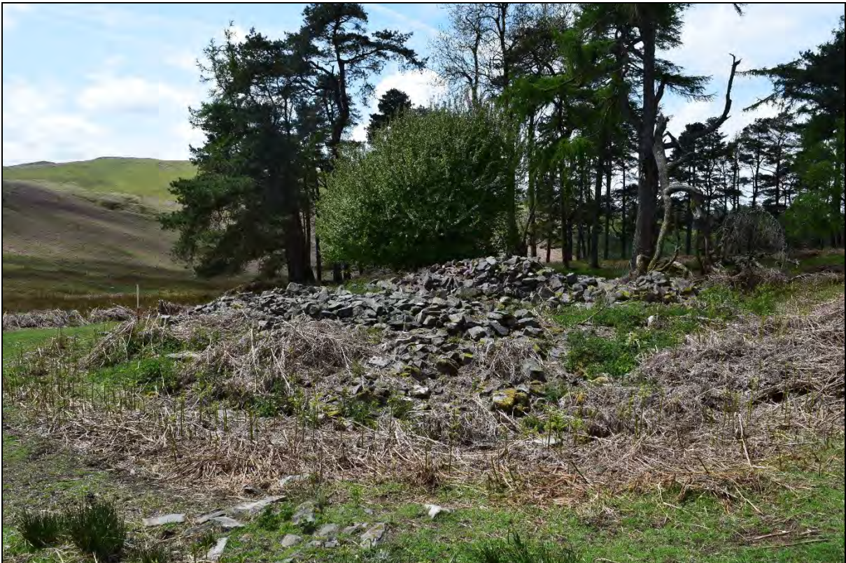
Plate 85: Rubble now marks the site of Birmingham Corporation's cottage at Ty'n y Pant (ID number 463), built circa 1900. Looking southwest.
