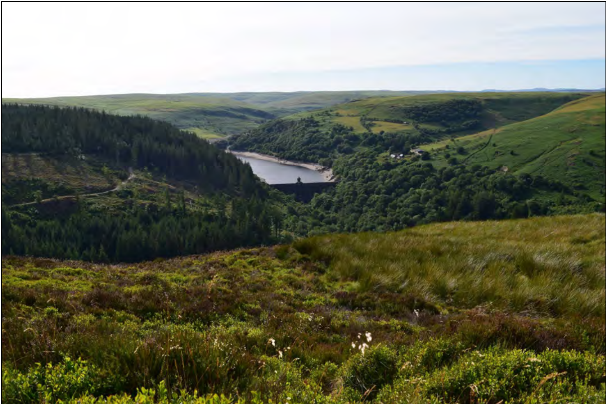
Plate 2: A view towards Penygarreg Dam at the heart of the Elan Links Survey Area. Penygarreg Farm is to the right of the dam. Looking west-northwest.
