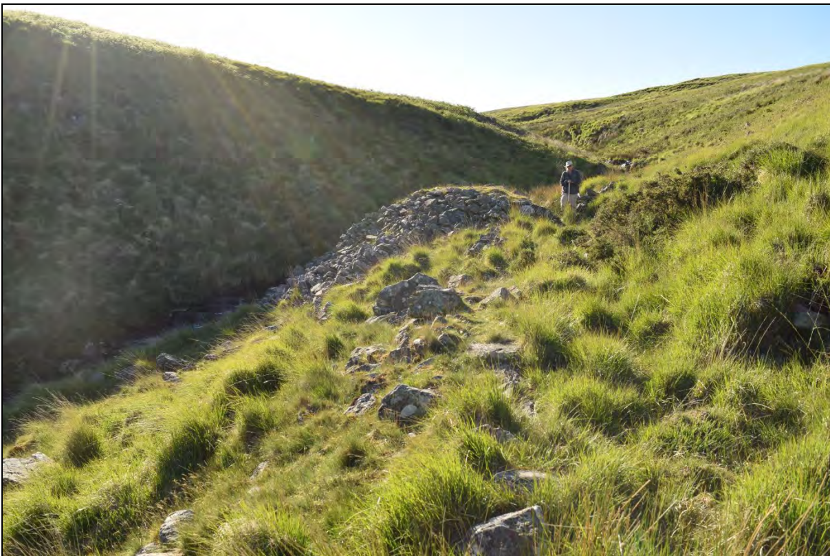
Plate 70: The Nant y Garw mine dam (ID number 573). Looking northwest.
