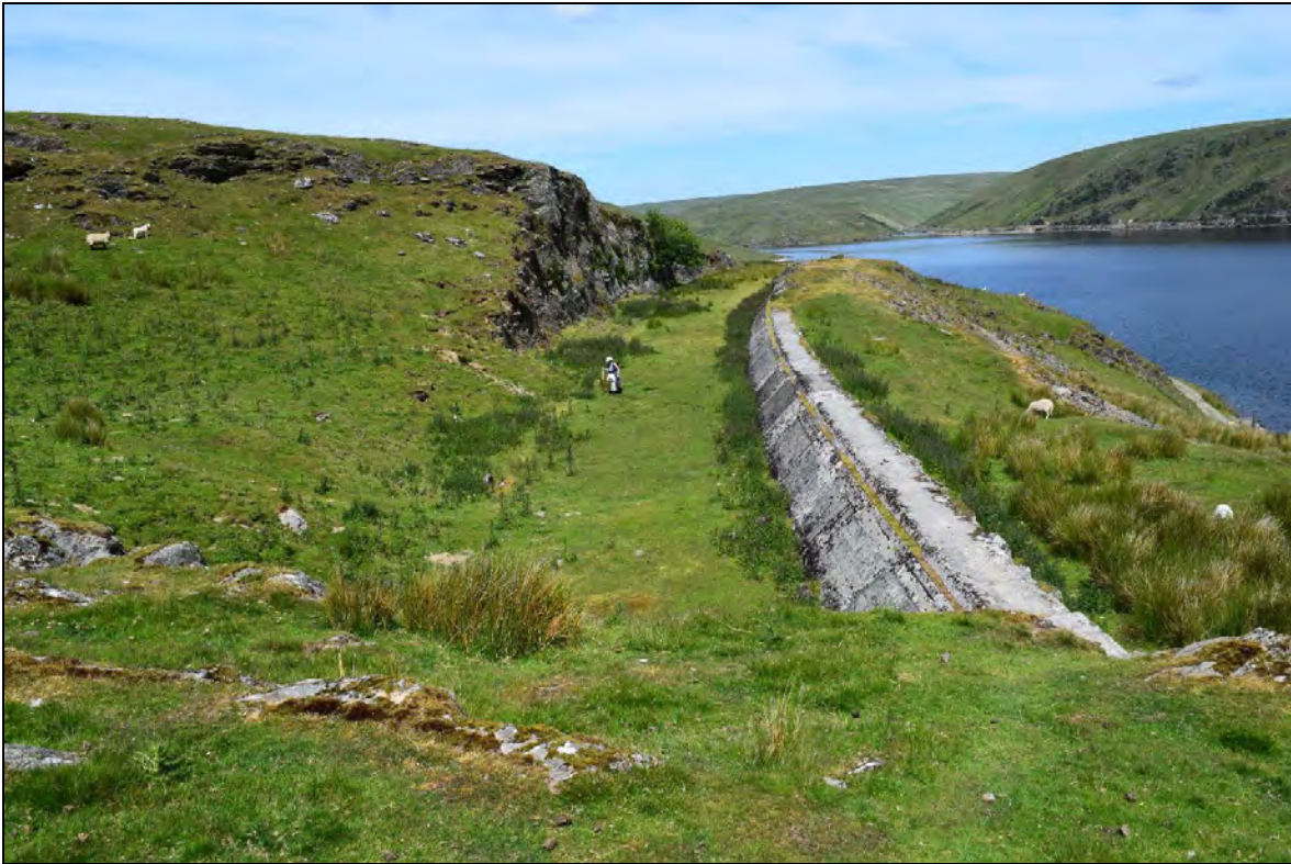
Plate 88: A quarried cutting fronted by a concrete and stone bund (ID Number 3314) to the western end of the Claerwen dam. Large cranes were mounted in the cutting during the construction period of the dam. Looking north-northwest.
