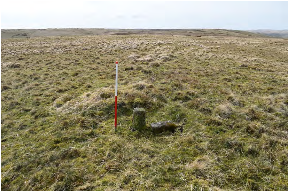
Plate 87: A broken concrete boundary marker near Penrhiw-wen (ID number 3038), built circa 1900. The stones have stood for over a century and need to be monitored and maintained or replaced where necessary. Looking southwest.
