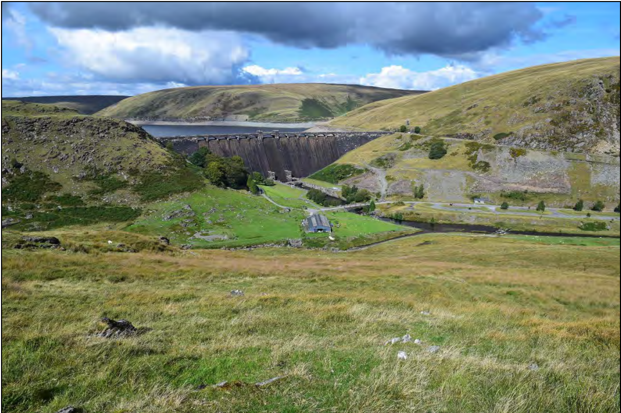
Plate 82: Claerwen Dam built in the mid-20 th century. Looking north.
