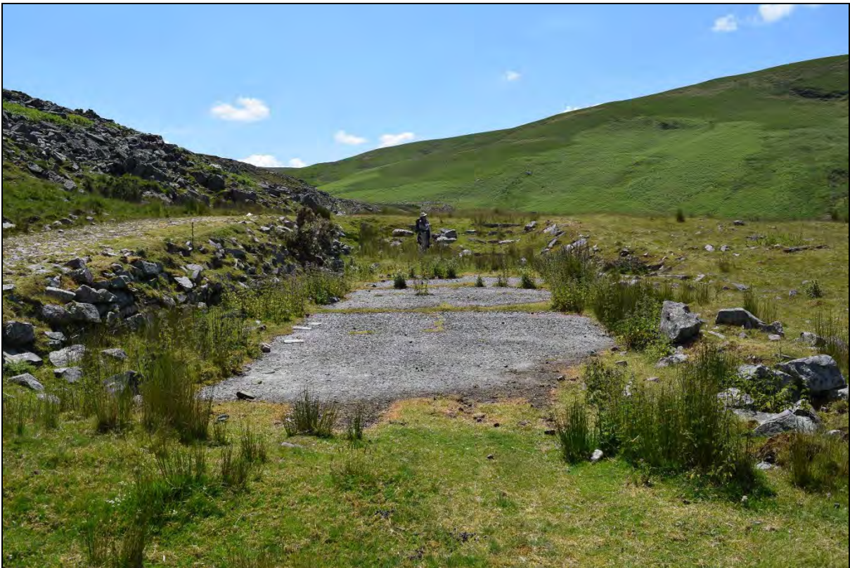
Plate 91: The concrete base of a quarry building (ID number 3326) at the Marchnant Quarry. Note the stone steps rising beyond the concreted area. Looking south-southwest.
