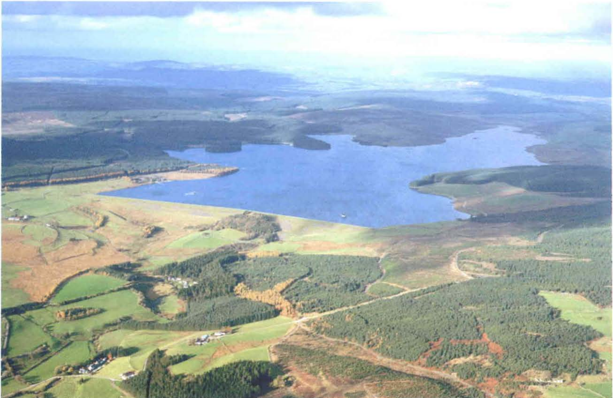
1112 Brenig Reservoir character area. Aerial view of Llyn Brenig from the south. The reservoir was constructed in the 1970s towards the eastern edge of Mynydd Hiraethog, flooding a medieval and later landscape of scattered farmsteads and fields. Photo: CPAT 01-C-152
