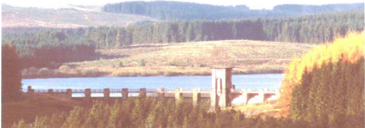
1111 Alwen Reservoir character area. The curved dam of concrete blocks with Italianate valve tower, viewed from the north-east. Photo: CPAT CS01/29/08
