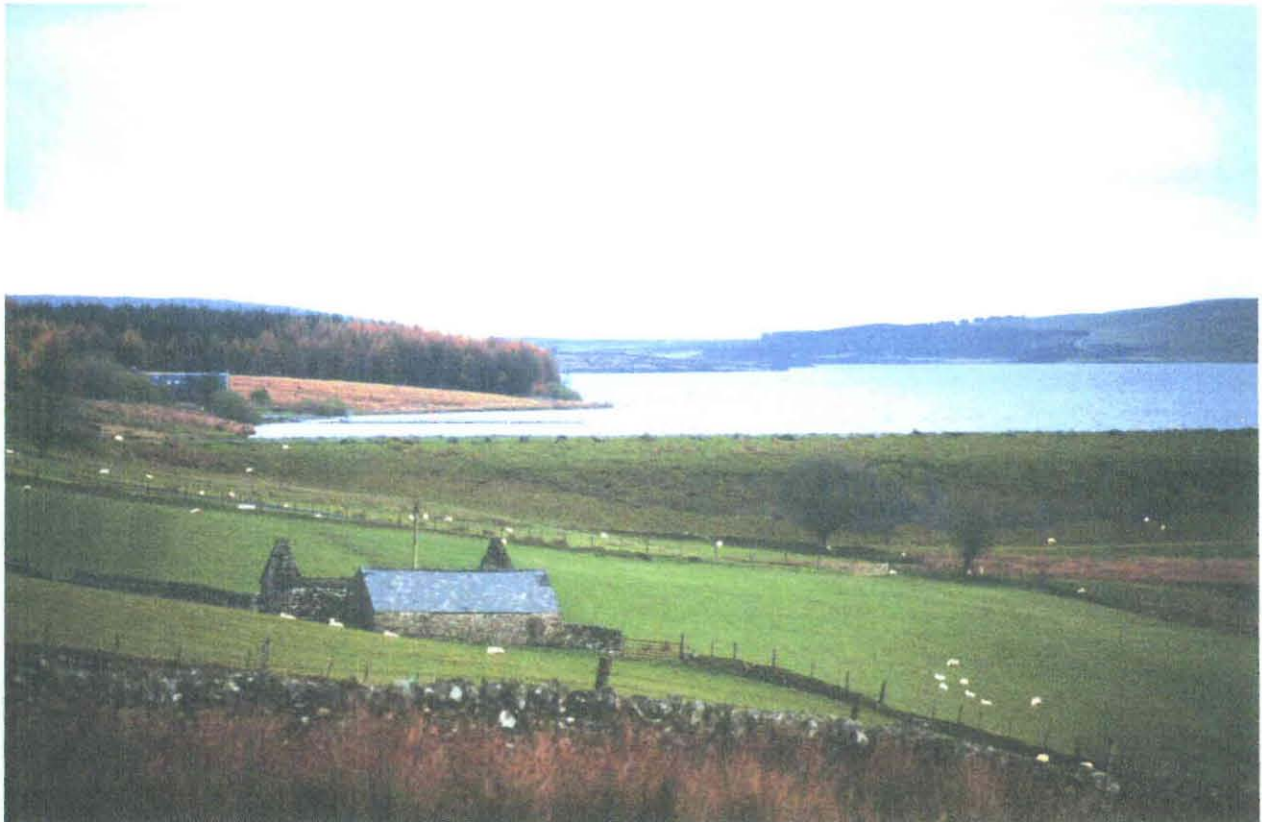
1112 Brenig Reservoir character area, with part of the farmstead of Elorgarreg Uchaf in the foreground. The construction of the reservoir by means of a large earthen dam, across the broad valley of the Afon Brenig and Afon Fechan, is in marked contrast to the earlier 20th-century reservoirs on Mynydd Hiraethog, characterised by the Aled Isaf and Alwen reservoirs, constructed by means of curved concrete dams set across much narrower valleys. Photo: CPAT CS01/29/13
