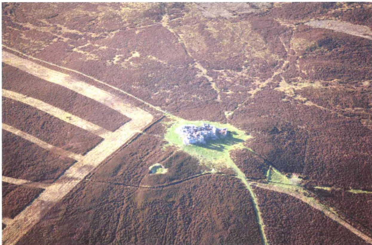
1107 Moel Bengam character area. Aerial view of the ruins of Gwylfa Hiraethog on Bryn Trillyn, to the west of the Sportsman's Arms. The building, one of the important landmarks on Mynydd Hiraethog, was built as a shooting lodge in 1913 by the entrepreneur Hudson Ewbanke Kearley but has been largely uninhabited since 1925. The roof survived into the 1970s but only some of the walls now remain as a testament to a former age. Photo: CPAT 01-C-190
