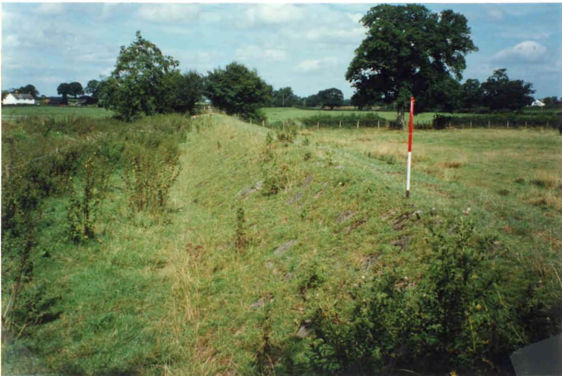
Plate 8 New Cut Argae at SJ 25471441, showing armouring of bank, from south-west
