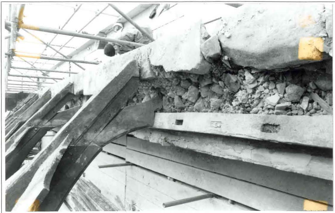
Plate 5 South Aisle roof showing brick infill by truss 3. Photo CPAT 944.12A
