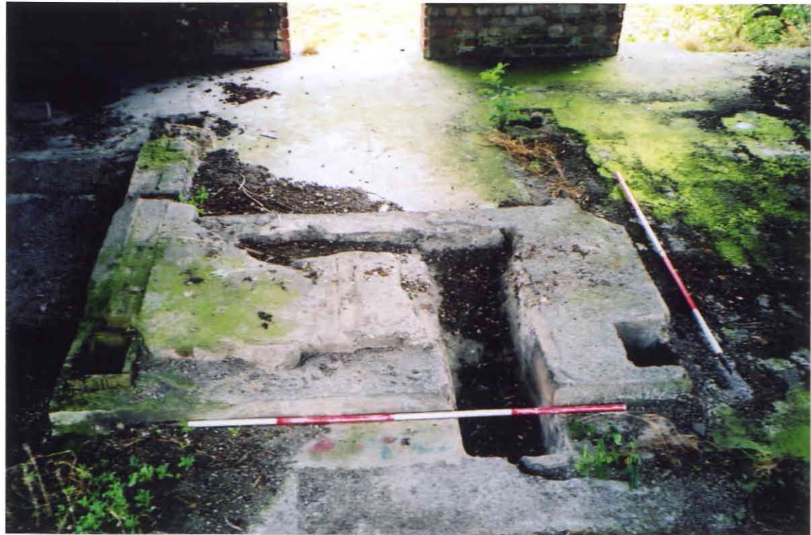
Plate 3 Machine base for winding gear. Photo CPAT 1077.19
