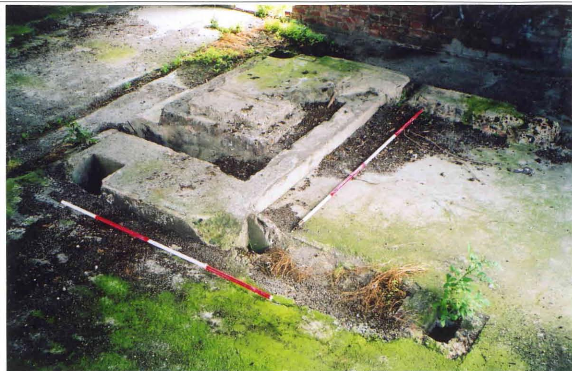
Plate 4 Machine base for winding gear. Photo CPAT 1077.23
