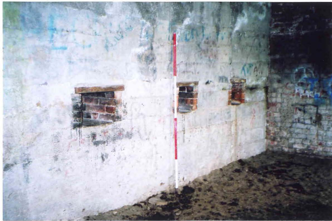
Plate 1 Ground floor: concrete support for winding gear. Photo CPAT 1077.16
