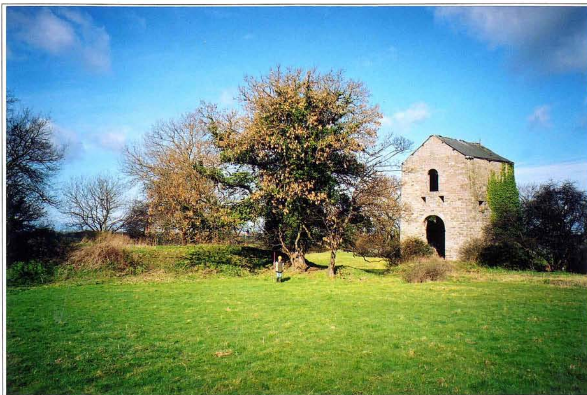
Plate 9 Clive Engine House and Winding Shaft from SE. Photo CPAT 1158.05
