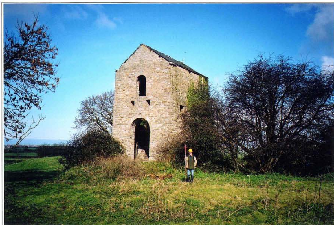
Plate 10 Winding Engine base from SE. Photo CPAT 1158.07
