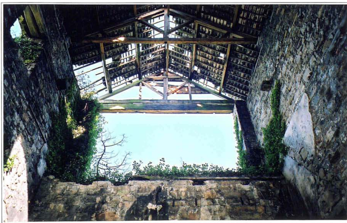
Plate 6 Clive Engine House: interior of north, bob-wall and roof. Photo CPAT 1158.17
