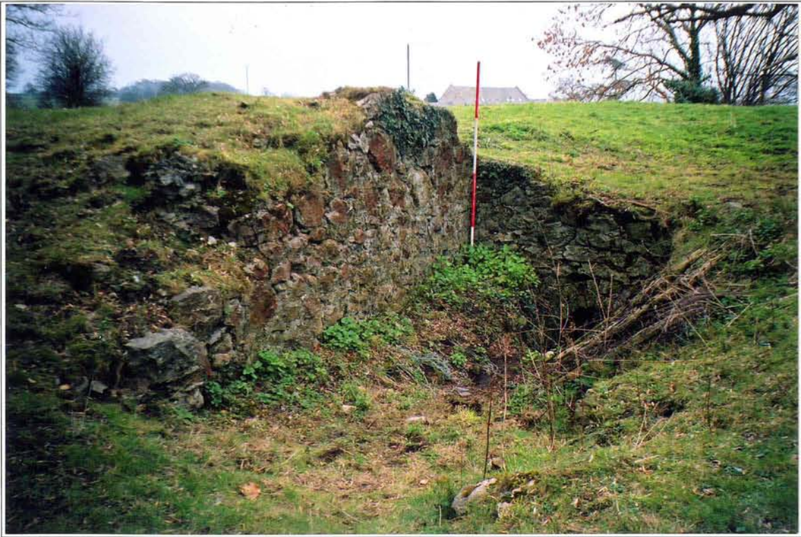
Plate 7 Culvert W of engine house from NE. Photo CPAT 1159.12
