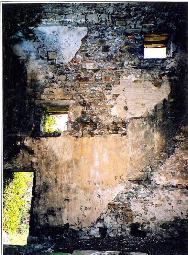
Plate 5 Clive Engine House: interior E wall showing position of stairs. Photo CPAT 1158.12
