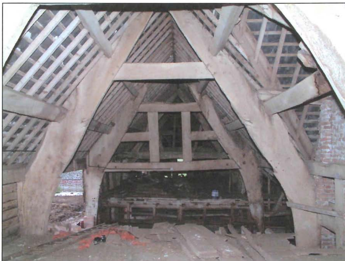
Plate 9 Barn 3 crucks, Trusses 2 and 3. Photo CPAT 1682.84
