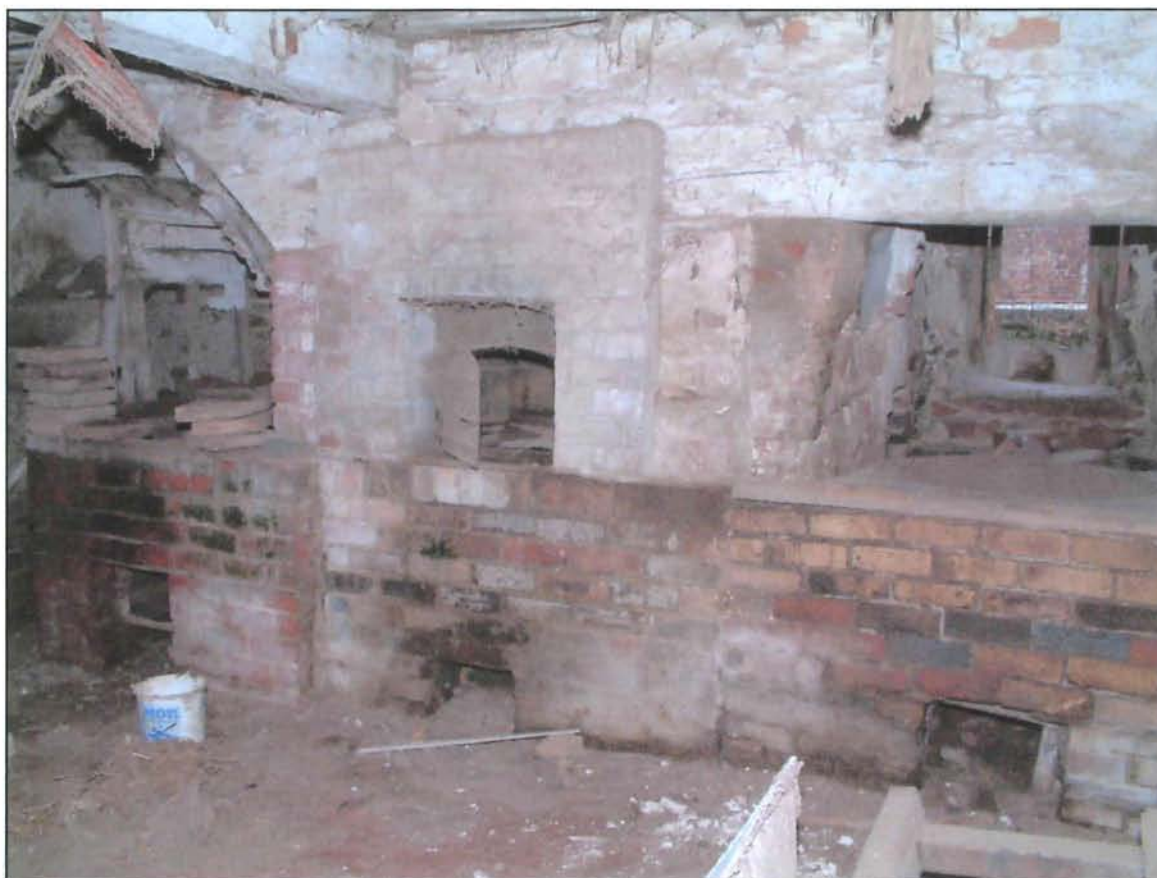
Plate 5 Barn 2 room G1, oven and boilers. Photo CPAT 1682.27
