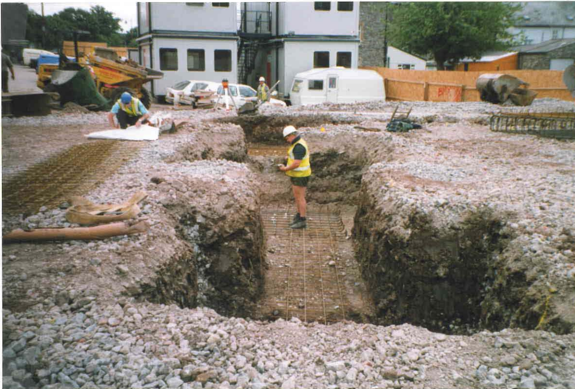
Plate 3 Foundation trench excavation for retail store. Photo CPAT 843.17
