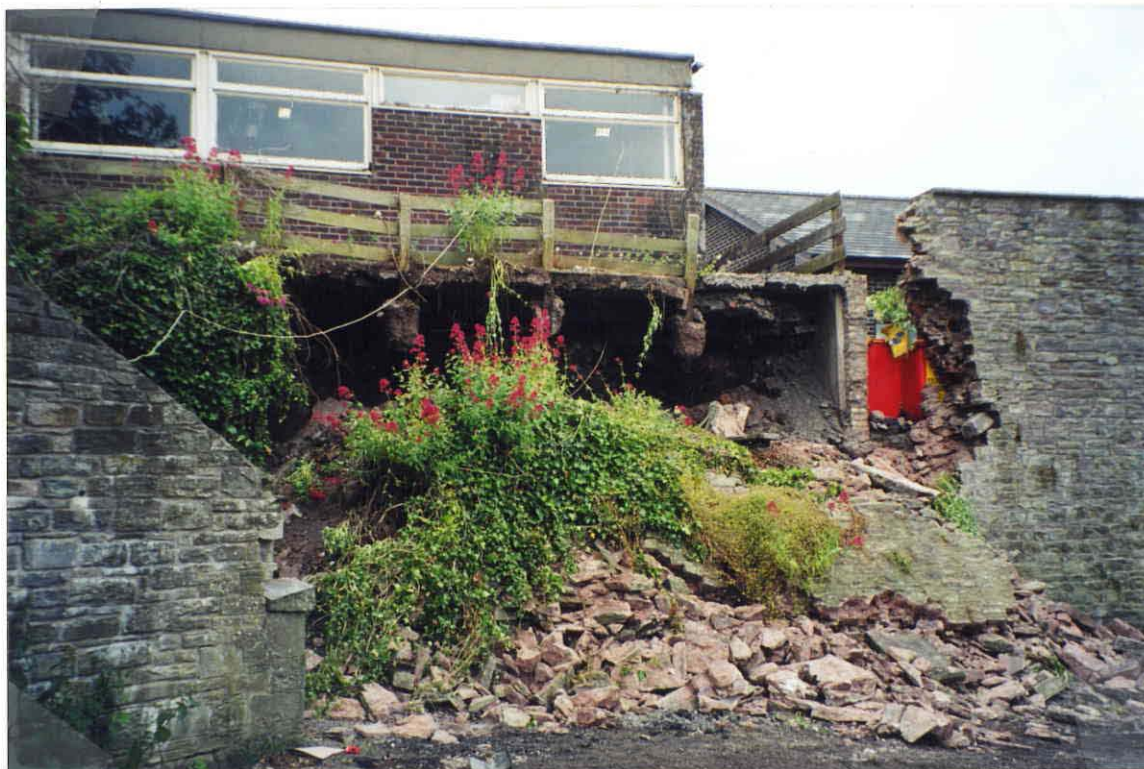
Plate 1 Collapsed section of boundary wall from NE. Photo CPAT 824.1
