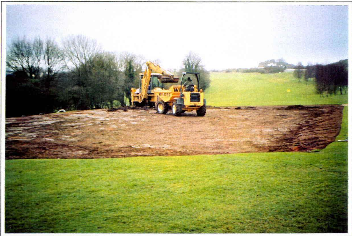
Plate 1 Mechanical stripping of sand/peat make-up (1). Photo CPAT 1134. 24
