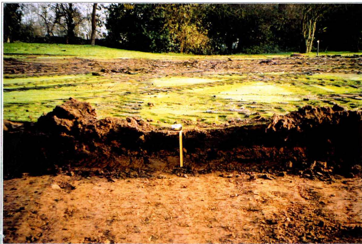
Plate 3 4th Green showing sand and peat make-up. Photo CPAT 1131.13
