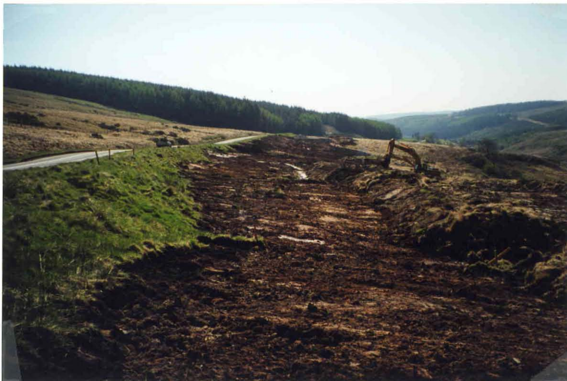
Plate 1. Topsoiling operations across area of common land. View from N. Photo CPAT 817.8
