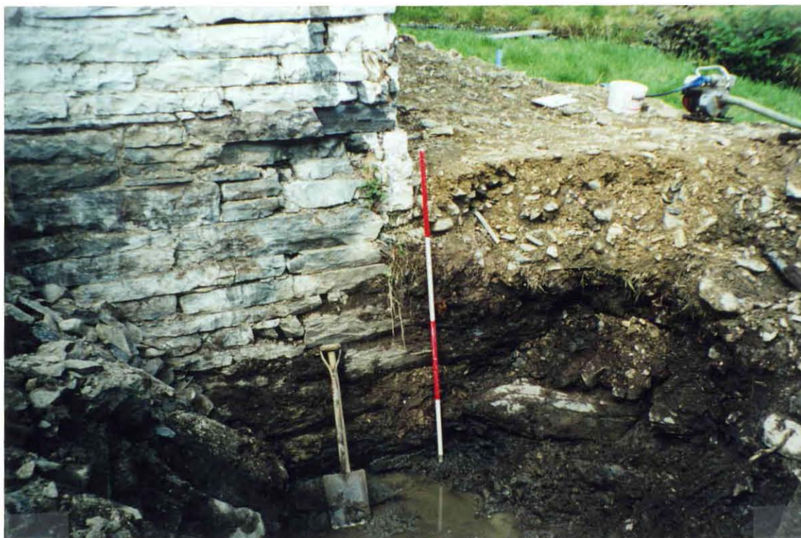
Plate 5 NE end of wheel pit and tailrace from SE. Photo CPAT 837.12
