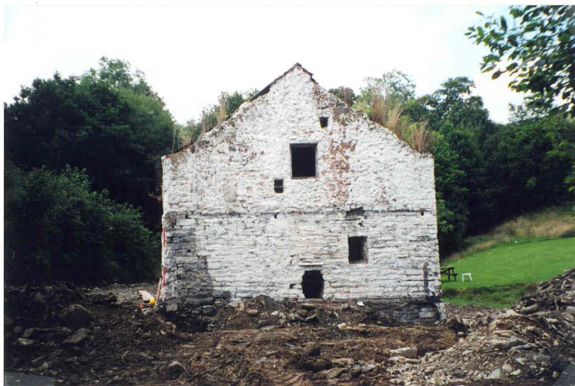
Plate 2 Mill house SE wall showing axle tree arch. Photo CPAT 837.5
