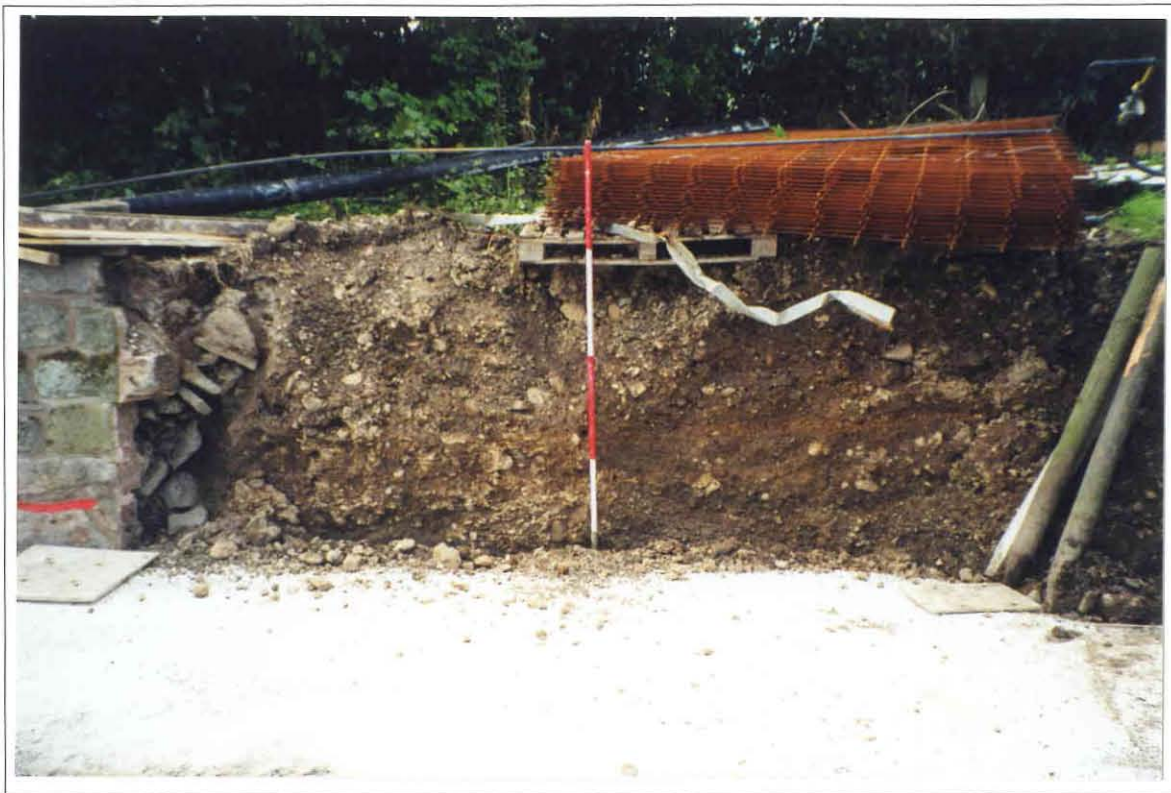
Plate 1 Collapsed section of bank adjacent to retaining wall. Photo CPAT 997.17
