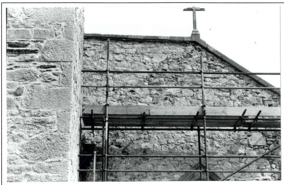
Plate 8: masonry infill on top of west wall of south nave
