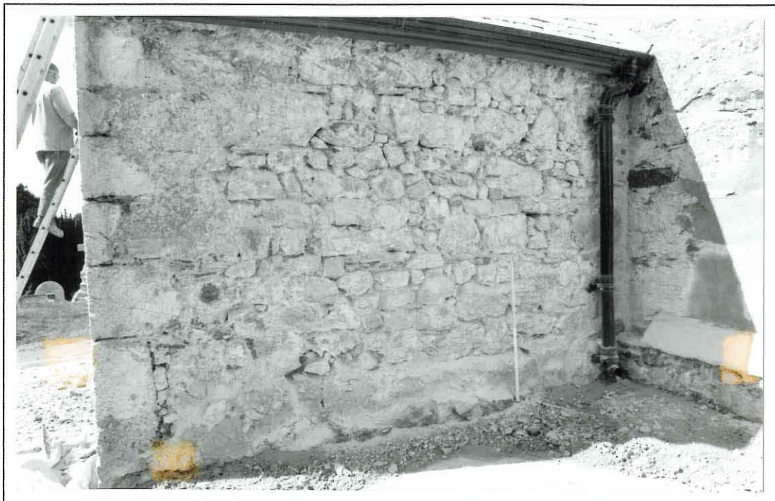
Plate 10: east wall of porch after render removal
