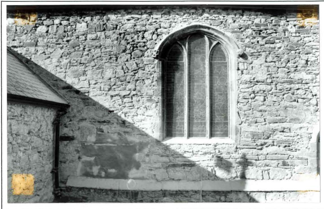
Plate 13: west window in south wall with decorated fragments above and to one side
