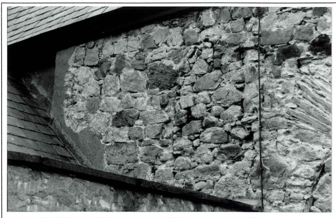
Plate 7: blocked window in north wall of north nave
