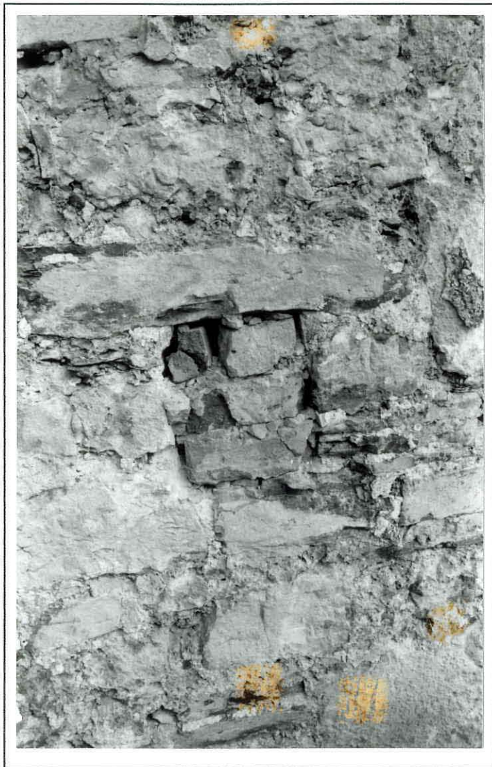
Plate 9: putlog hole in west wall of south nave
