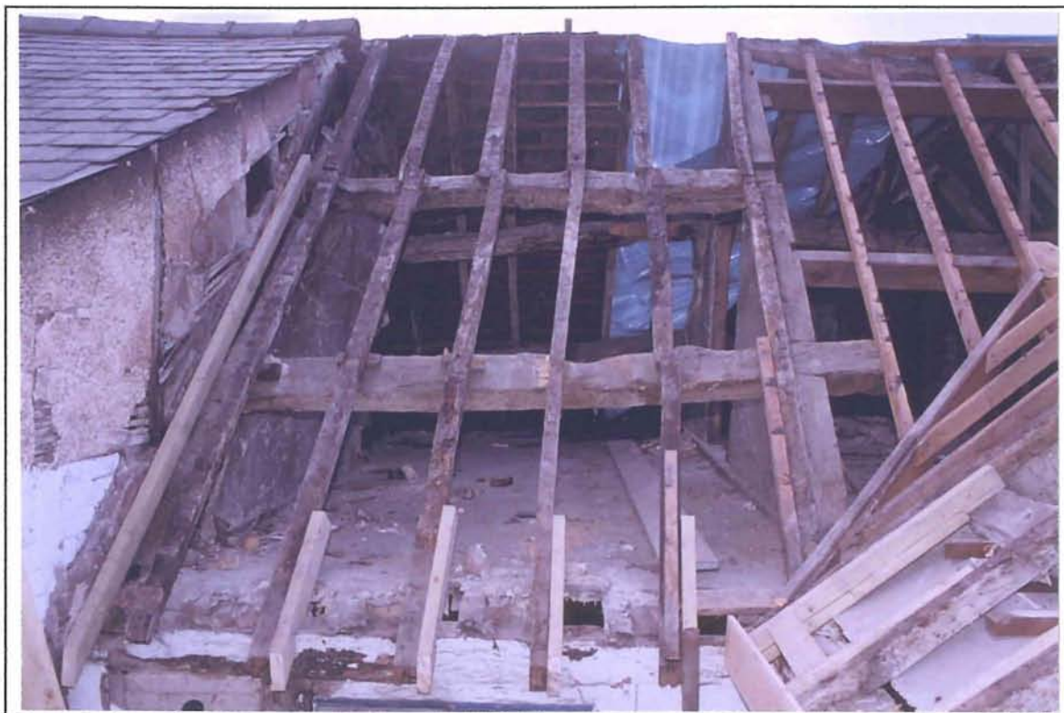
Plate 1 Main roof showing purlins cut for addition of porch. Photo CPAT cs04/06/20
