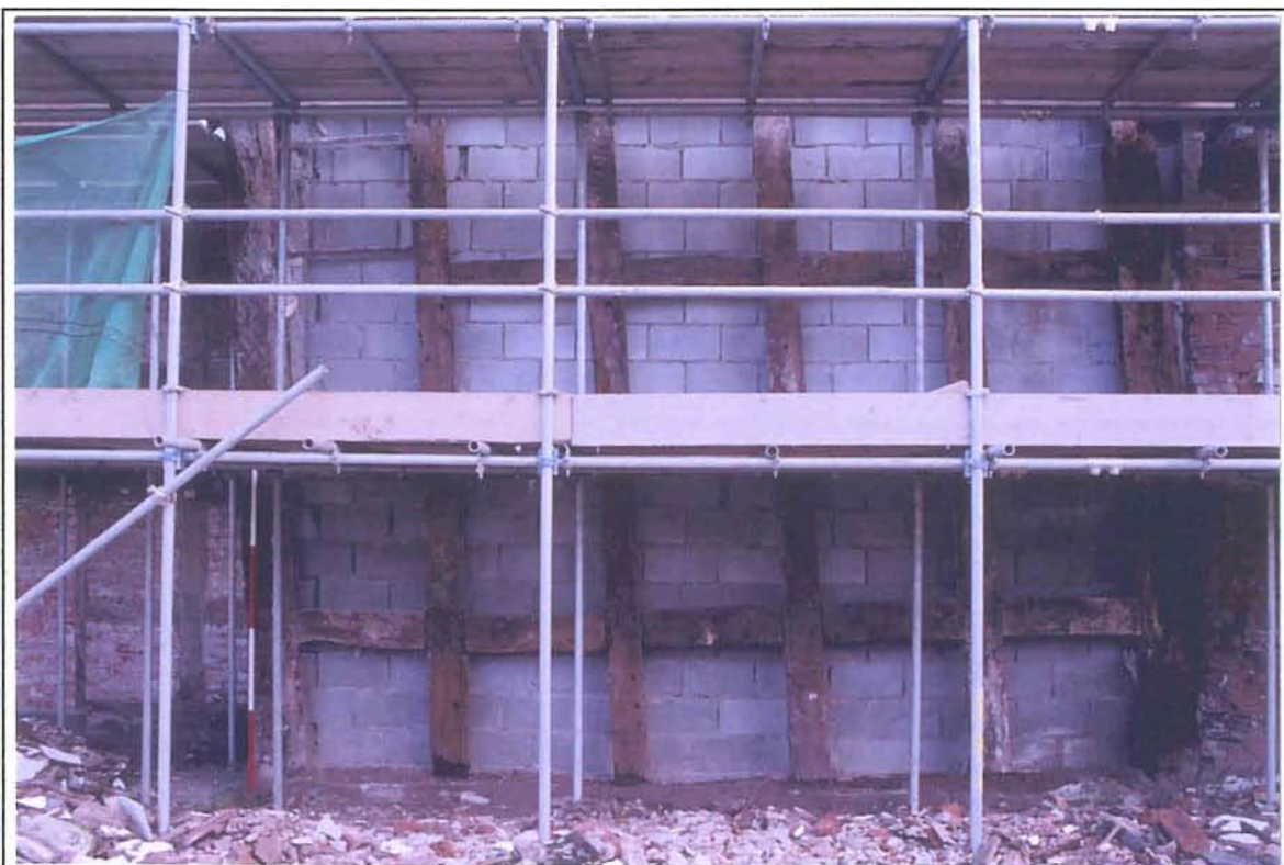
Plate 4 West elevation: open framing for main gable end wall. Photo CPAT cs04/05/04
