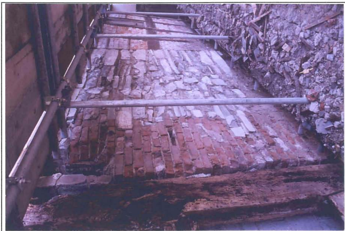
Plate 5 West elevation: rear wing showing stone and brick timber with timber framing beyond. Photo CPAT cs04/05/21
