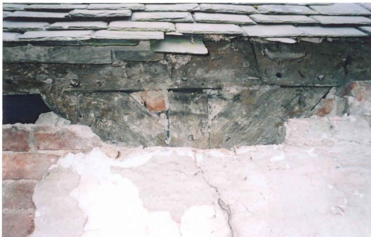
Plate 6 Truss 3 north wall-post / wall plate, from the north. Photo CPAT 1344.27
