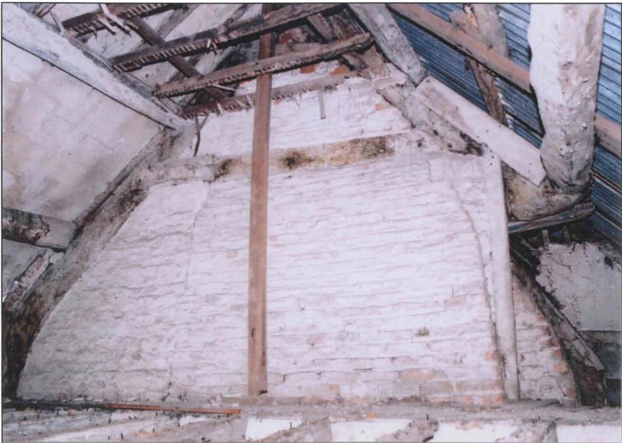
Plate 4 Truss 1 and the inserted 17th-century chimney structure, from the east. The truss was truncated on the right to allow for the stair. Photo CPAT 1343.22
