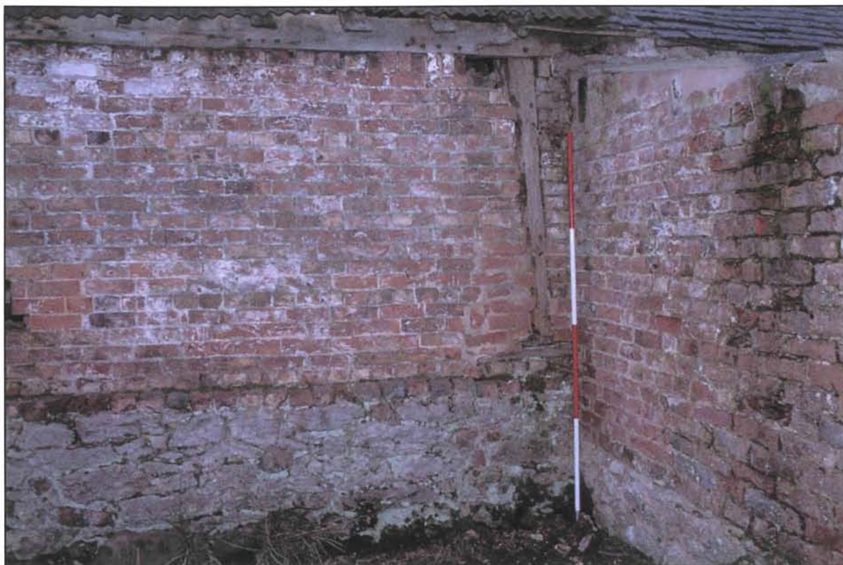
Plate 5 Truss 2 wall-post / wall plate adjacent to the 19th-century outhouse, from the north. 2m scale. Photo CPAT CS03/24.11
