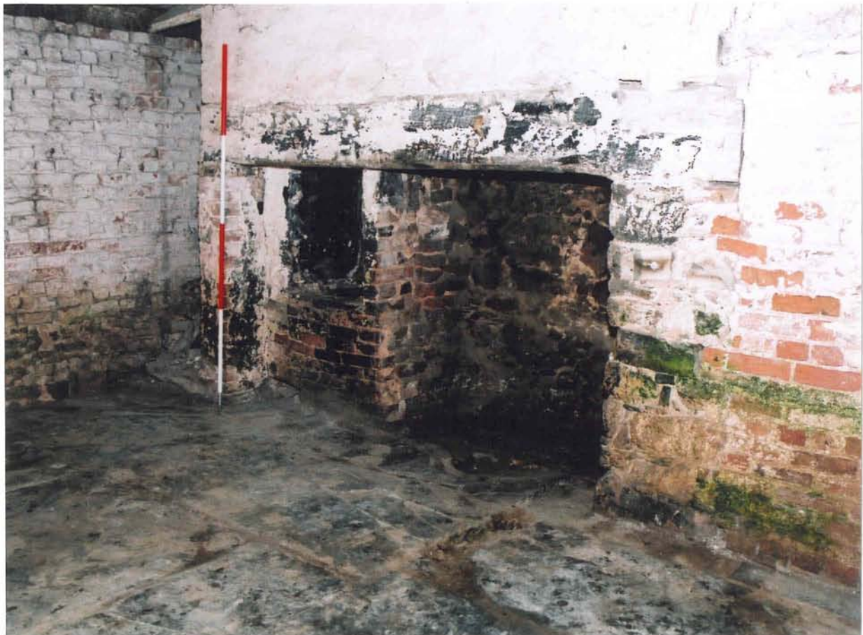
Plate 2 West side of the 17th-century fireplace and the slate slab floor. To the left of the fireplace is access to the later stair, while on the right is the blocked doorway. 2m scale. Photo CPAT 1343.16
