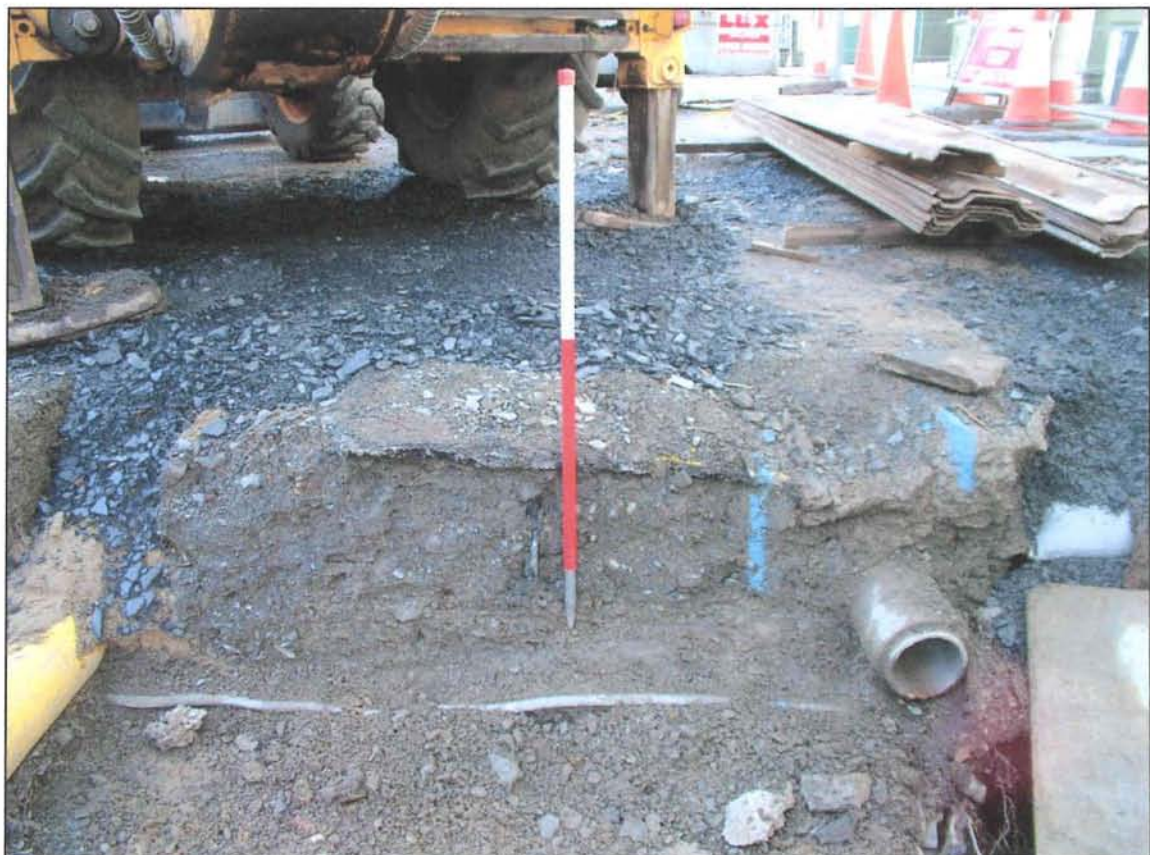
Plate 2 Southern section showing former cobbled road surface (at base of scale) with levelling material above.
