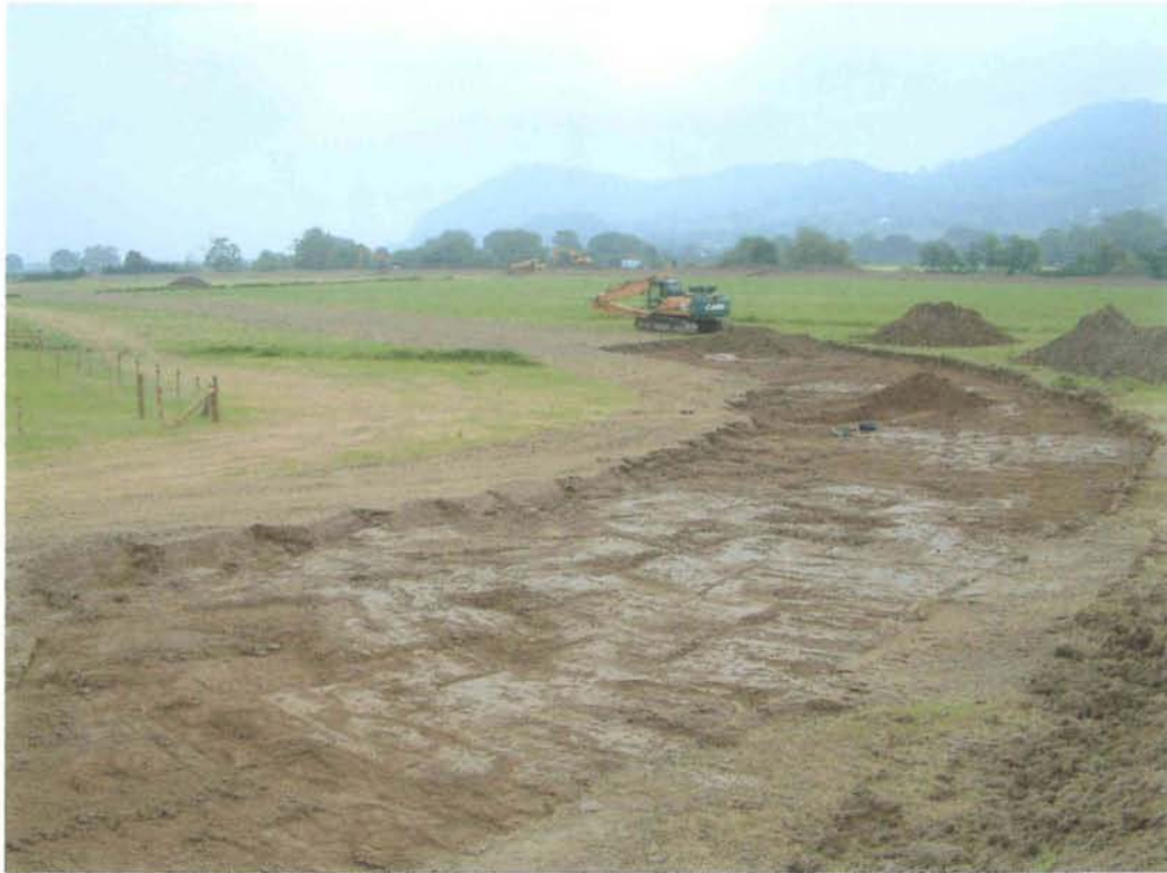
Plate 1: Topsoiling in preparation for the construction of the new argae.
