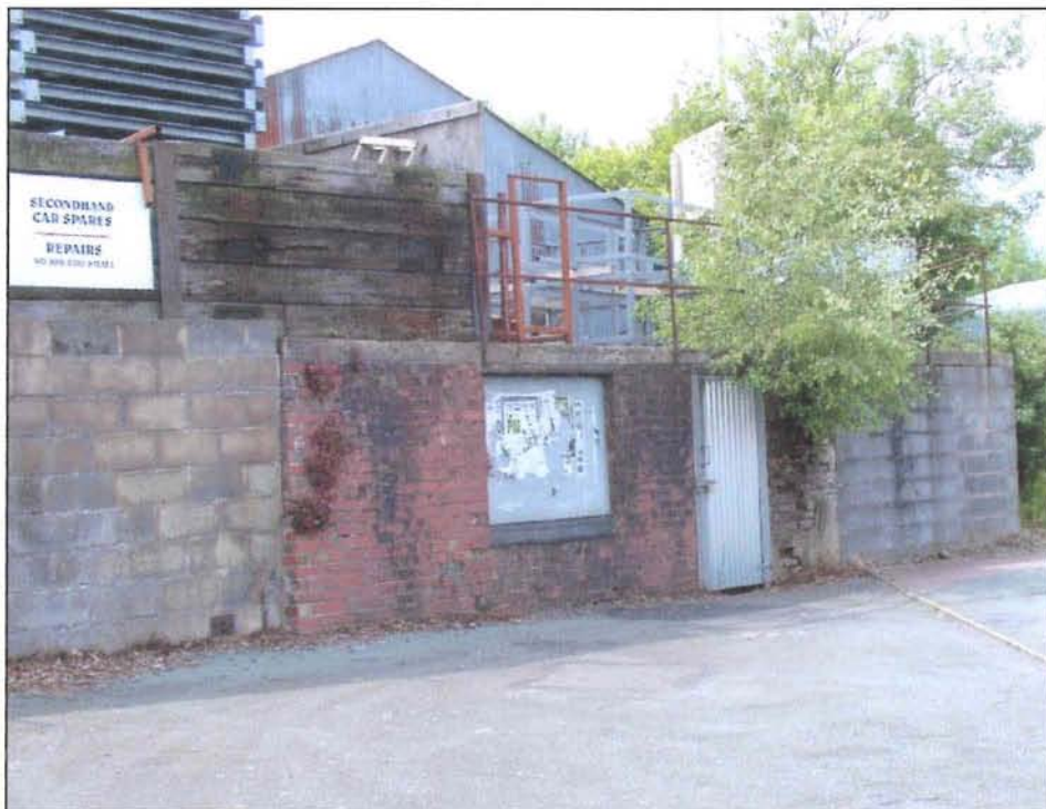
Plate 2 Site 5 from the north. Photo CPAT 2438-010
