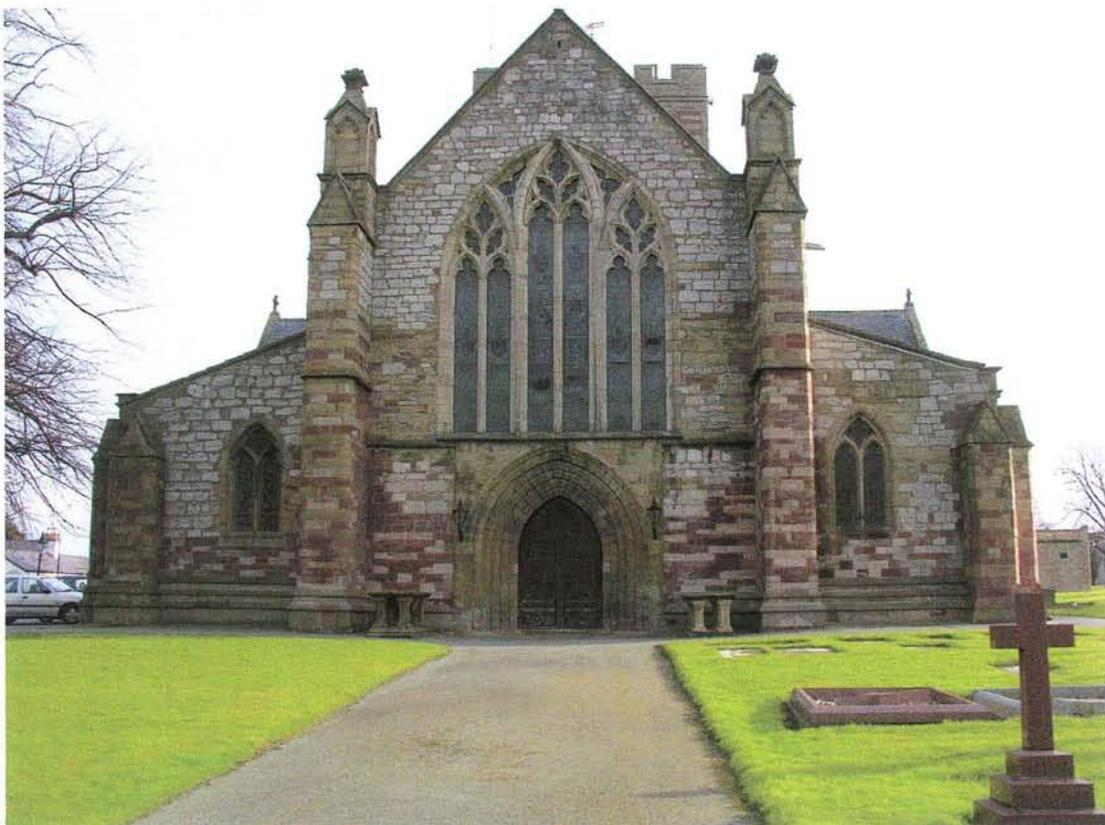
West wall: a truly heterogeneous fabric mix, with considerable colour variation, unmatched elsewhere in the cathedral. Seen from the side the wall has a slightly outwards lean at the gable apex. Three features: the west doorway, the big west window above it and a small slit immediately below the apex of the roof, in addition to which there are two buttresses.
