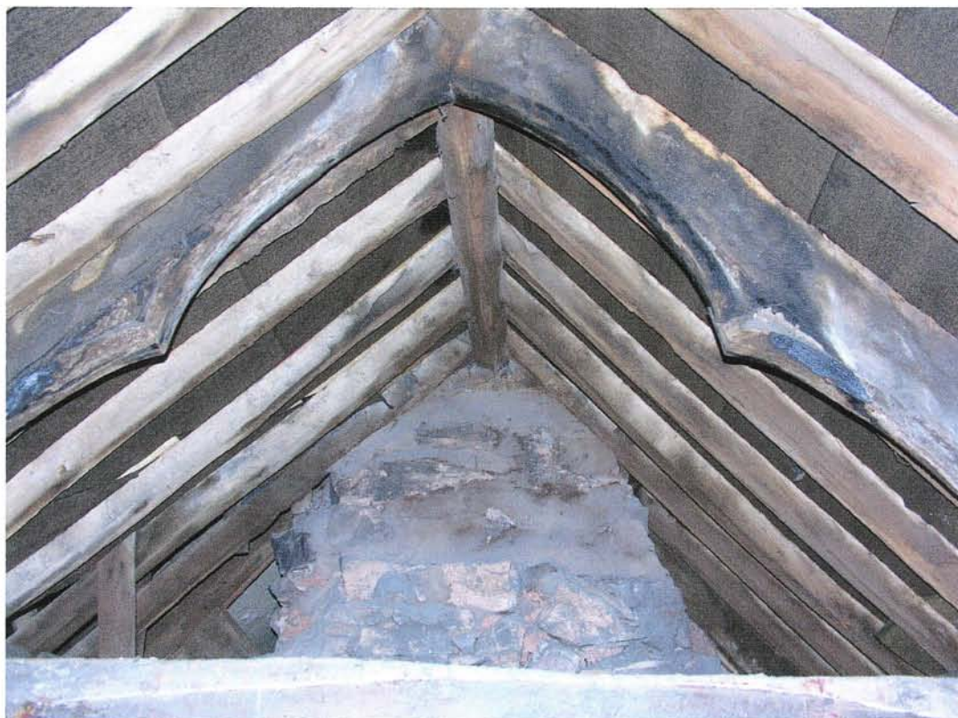
Fig. 6. Truss 1, upper part showing the cusped blades.
