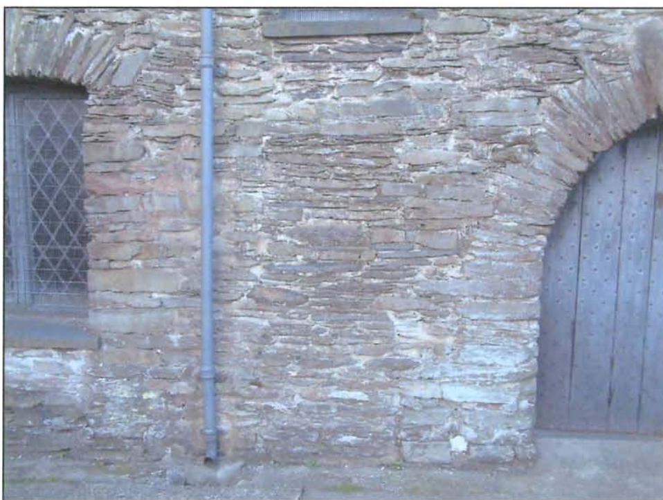
Plate 4 Blocked door in north elevation. Drain pipe marks location of rear wing (Photo CPAT 1694. 43)
