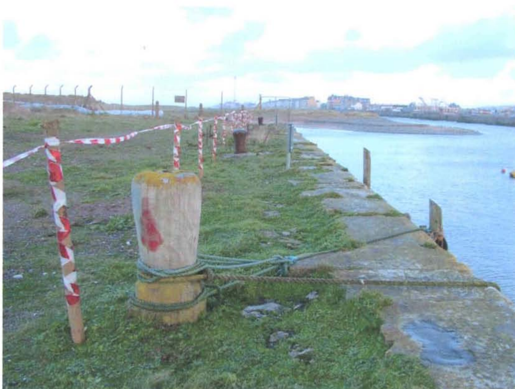
Plate 4 Mooring posts along the quayside. Photo CPAT 2301.001
