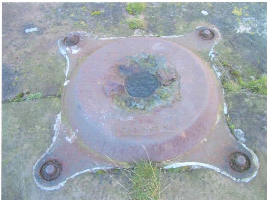
Plate 5. Cast iron crane base along quayside. Photo CPAT 2301.004
