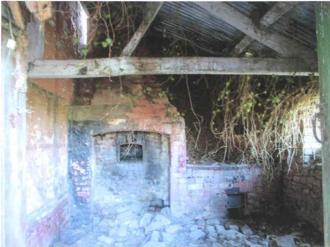
Plate 5 Oven with boiler to right
