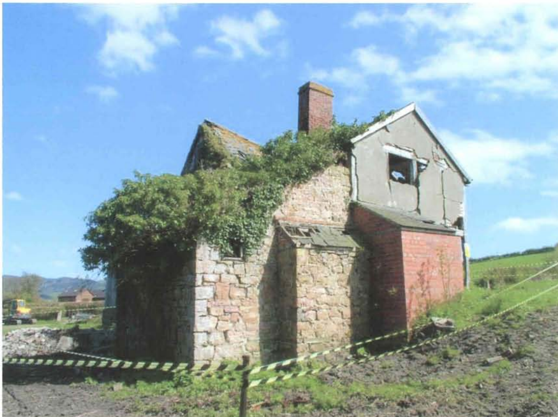
Plate 4 West elevation showing the projection for the oven and later brick privy
