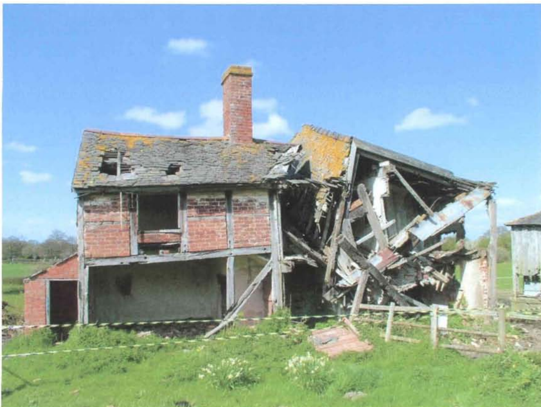
Plate 1 South elevation showing collapsed southern gable and later box-frame extension
