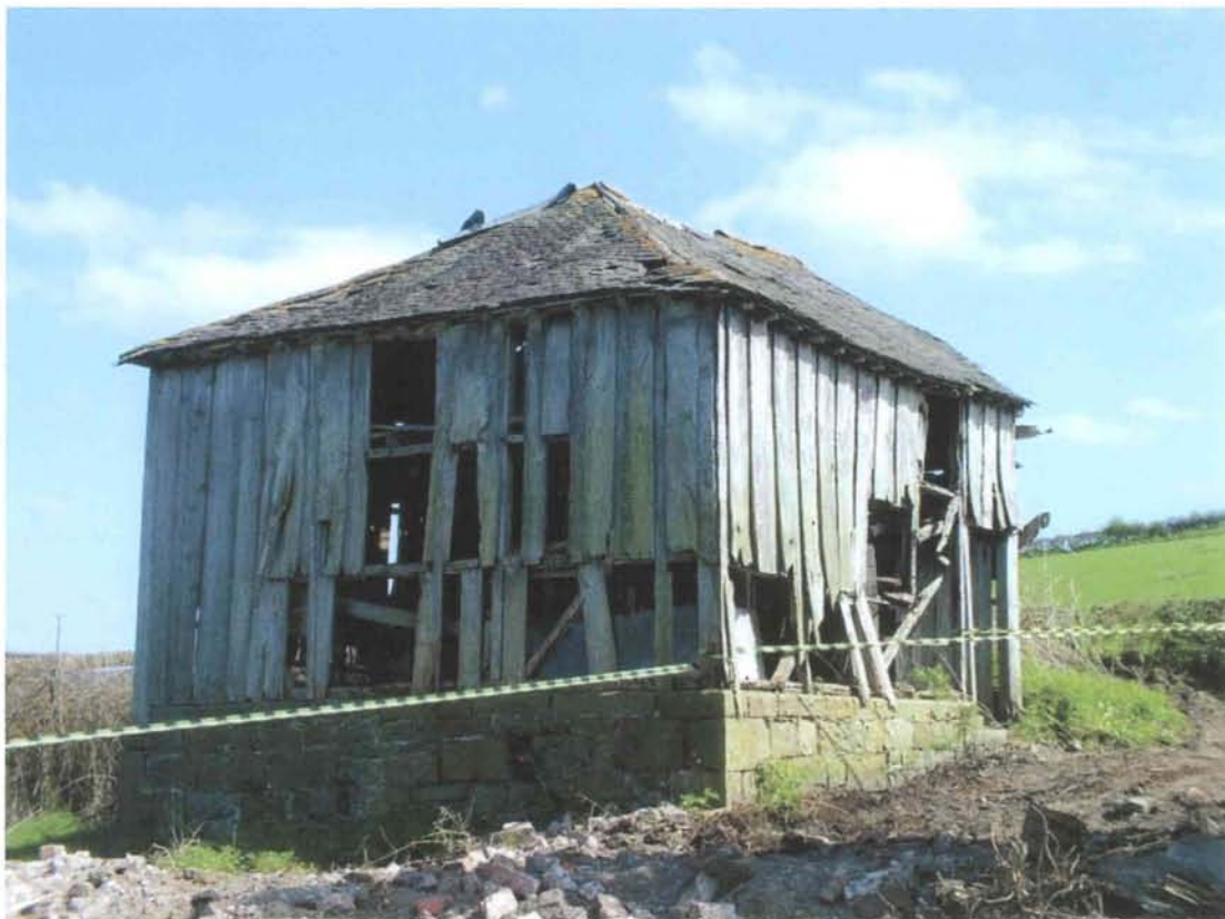
Plate 6 Barn viewed from north-west showing stone plinth and hipped roof
