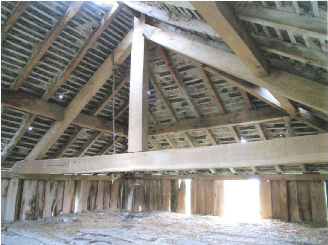
Plate 7 Barn first floor showing roof truss
