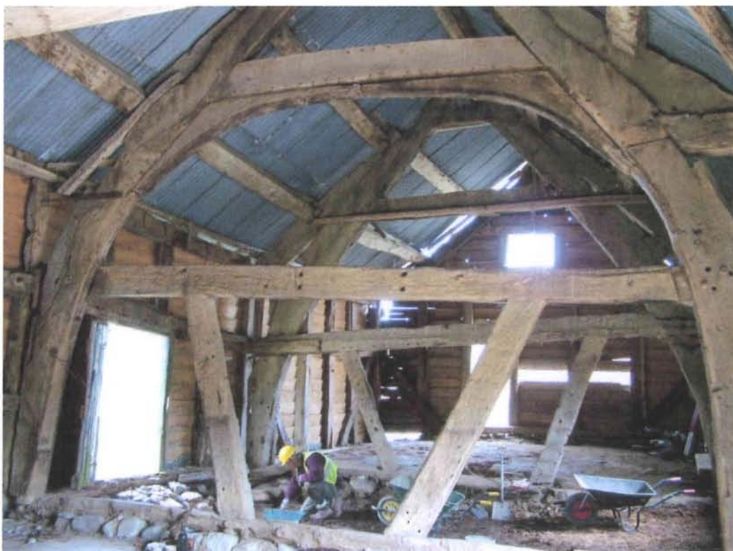
Plate 1 The central cruck of the hall from the west (CPAT Photo 2345-013)
