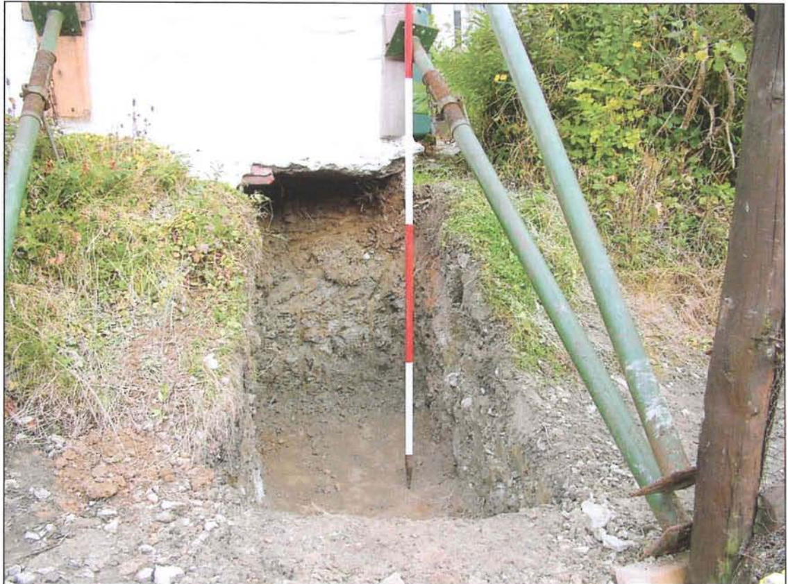
Plate 3 The trench excavated beneath the corner of the cottage prior to underpinning (Photo CPAT 2655-000)
