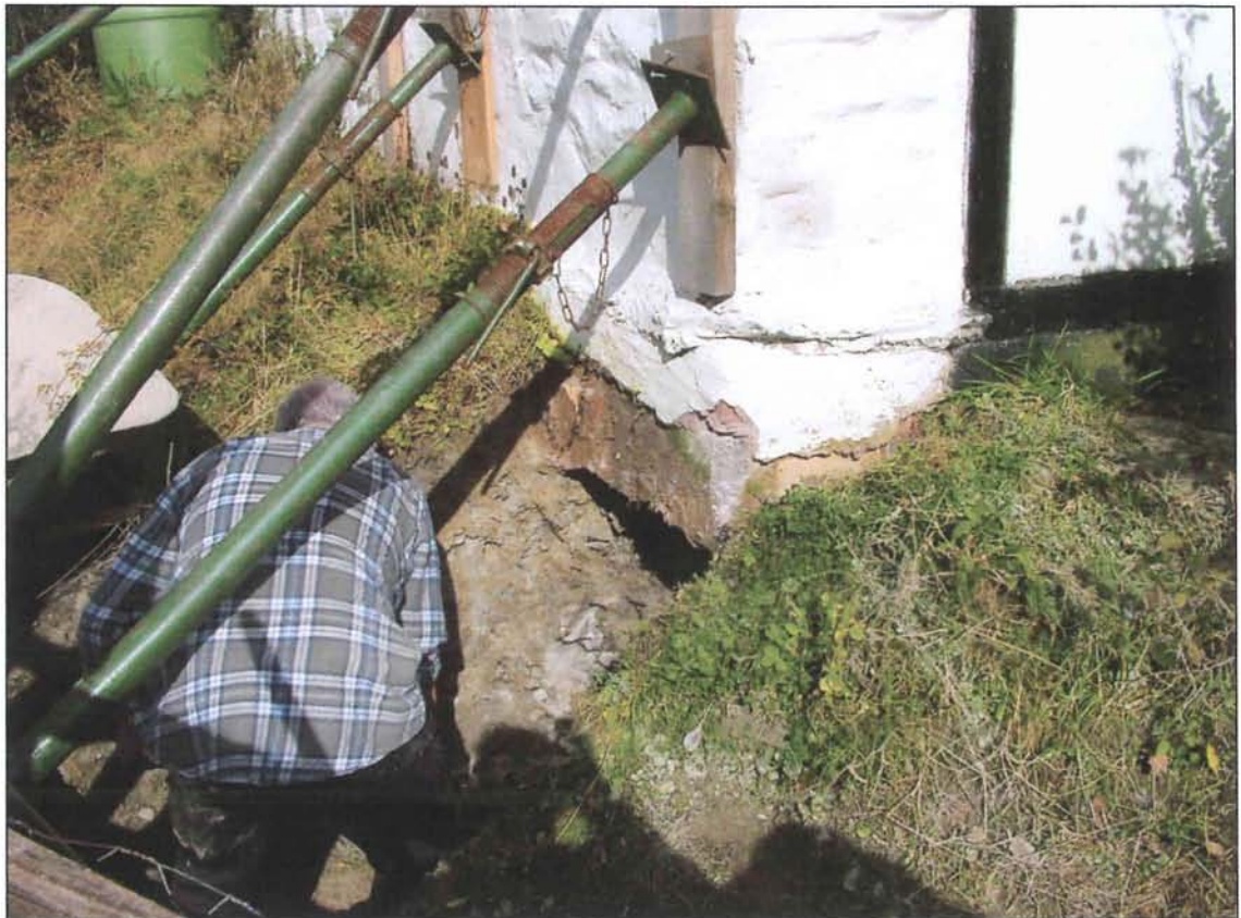
Plate 2 The corner of the cottage showing the previous attempt at underpinning beneath the original wall foundation (Photo CPAT 2655-000)
