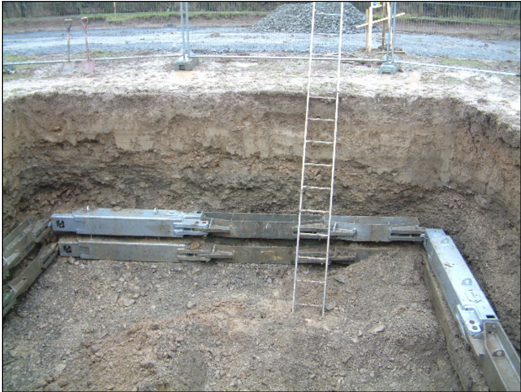
Plate 1 Test pit A viewed from the north-west
