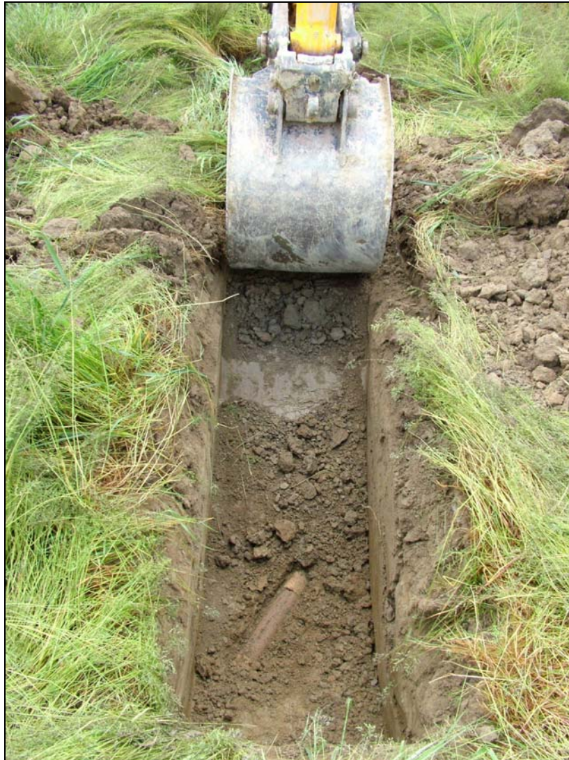
Plate 1 Sectional ceramic drainage pipes in the test pit at SJ 3271116070
