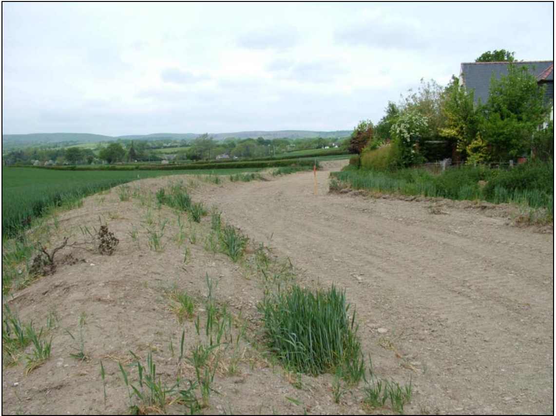
Plate 1: Section of topsoiled wayleave on the edge of Aberhafesp village, from south-east (Photo CPAT 3119-0002)
