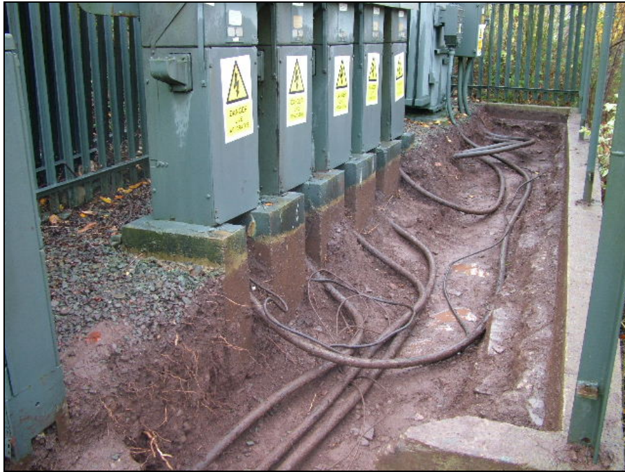
Plate 1. Excavation within sub-station compound. Photo CPAT 2980-004
