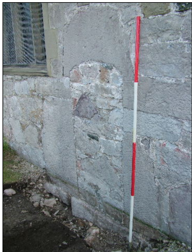
Fig. 21. The east doorway (Area D) with the modern drain removed from the base. Photo CPAT 2972-114.
