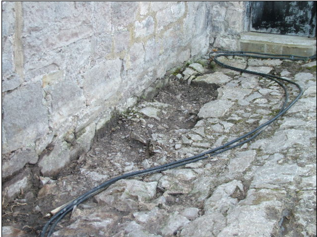
Fig. 7. Disturbance (31) in the vault roof alongside the nave wall. Photo CPAT 2972-043
