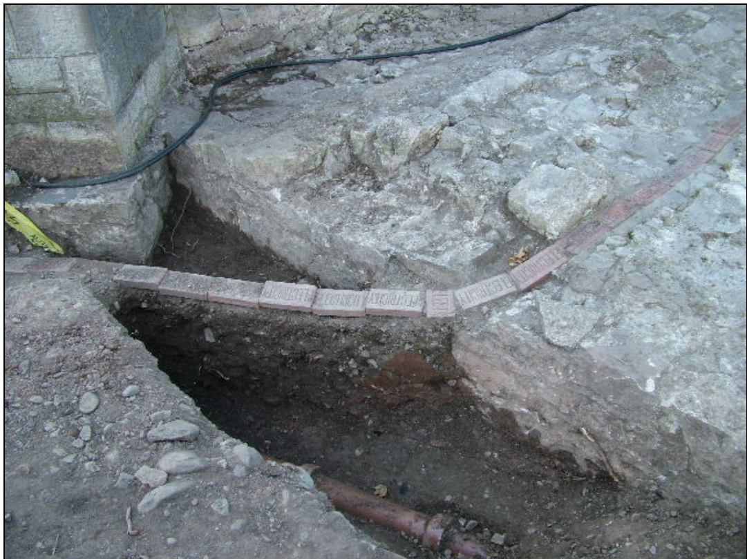
Fig. 9. Cable services and water drain (19) at east end of the vault. Photo CPAT 2972-035
