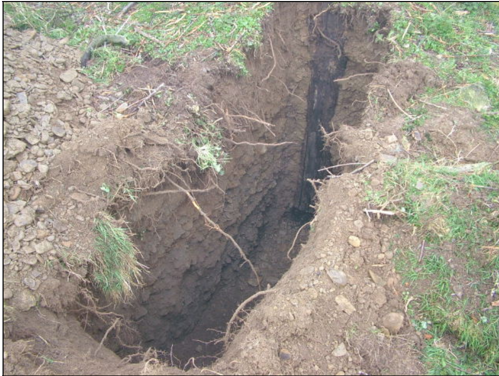
Fig. 3 Pit excavated for replacement electricity pole. Photo CPAT 2817.002
