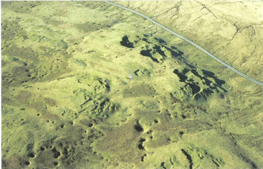
Aerial view of disused limestone quarry workings and limekilns just to the north of Cadair Fawr, viewed from the west in a landscape pitted with shake holes. In the right background is the main road (A4059) between Penderyn and Brecon, which originated as a turnpike road in the early 19th century. Photo: CPAT 08-C-71
