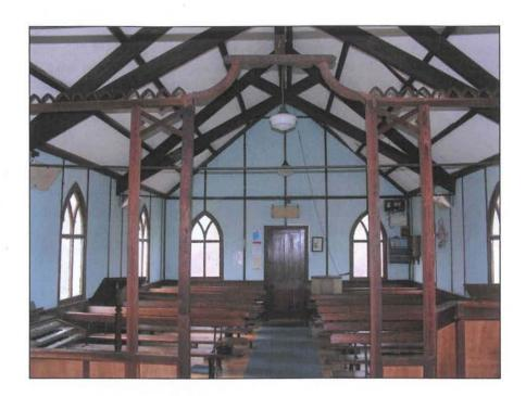
Internally, the roof is supported on three trusses with scissor supports and there is a panelled wooden floor, and walls of painted plyboard or similar. Each long wall has four two-light timber windows with Y-tracery and transoms, and there are two more at the west end, and a further one high up in the east wall.
