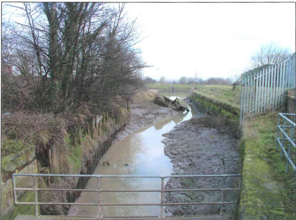
Fig. 16 Sandycroft Quay showing timber revetment on the left and stone revetment on the left.
