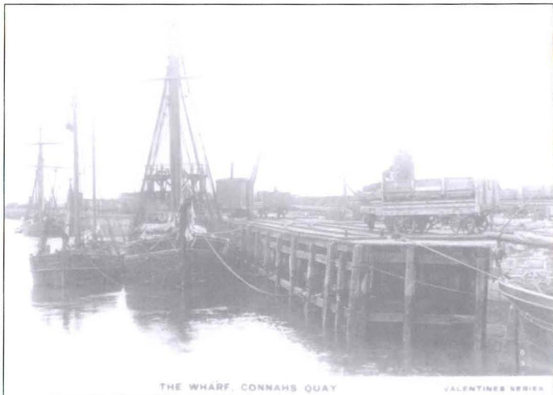
Fig. 3 Connah's Quay docks c. 1900 showing timber wharfage (PRN 83019) between Docks I and II. Note the steam crane on the dockside and the wagon on a turntable.
