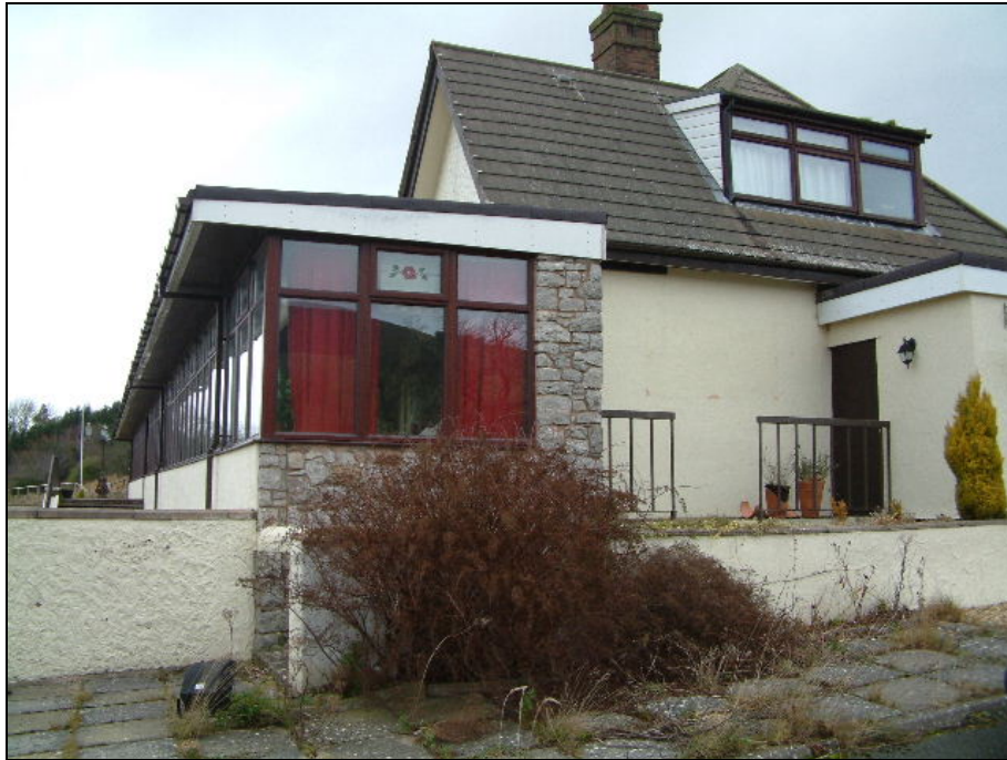
Figure 4. View of Clwyd Gate Restaurant from the south-east. (Photo CPAT 2700-004).
