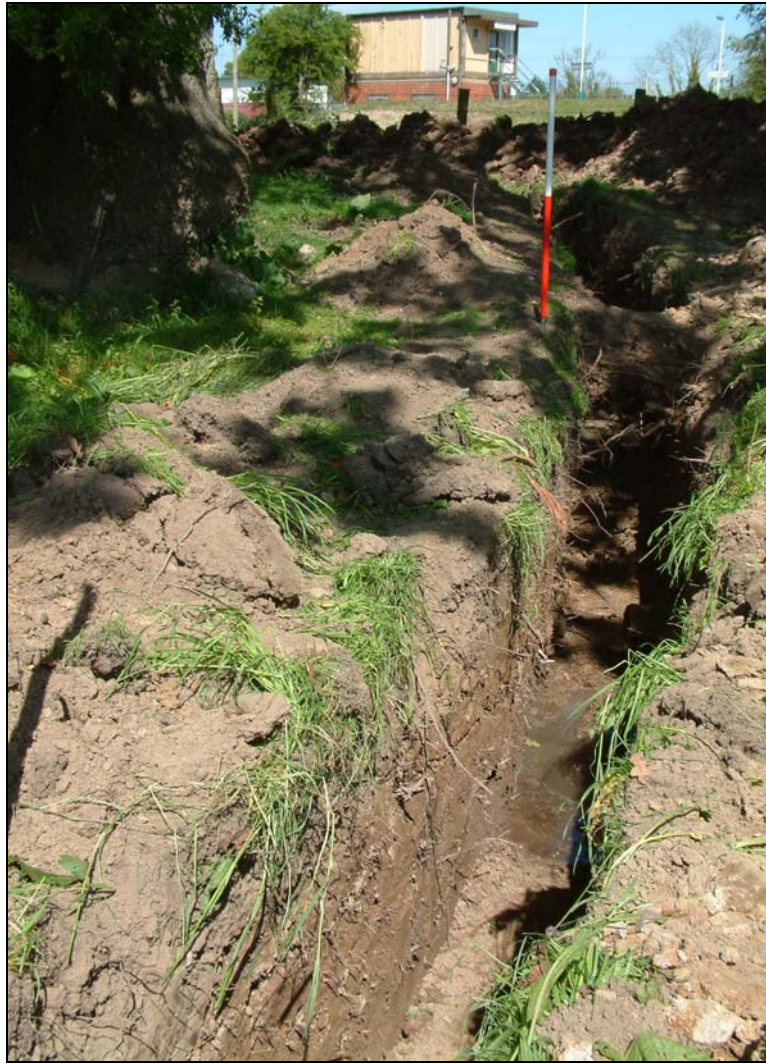
Plate 3 South-facing section of pipe trench showing upper ditch silts (3)
