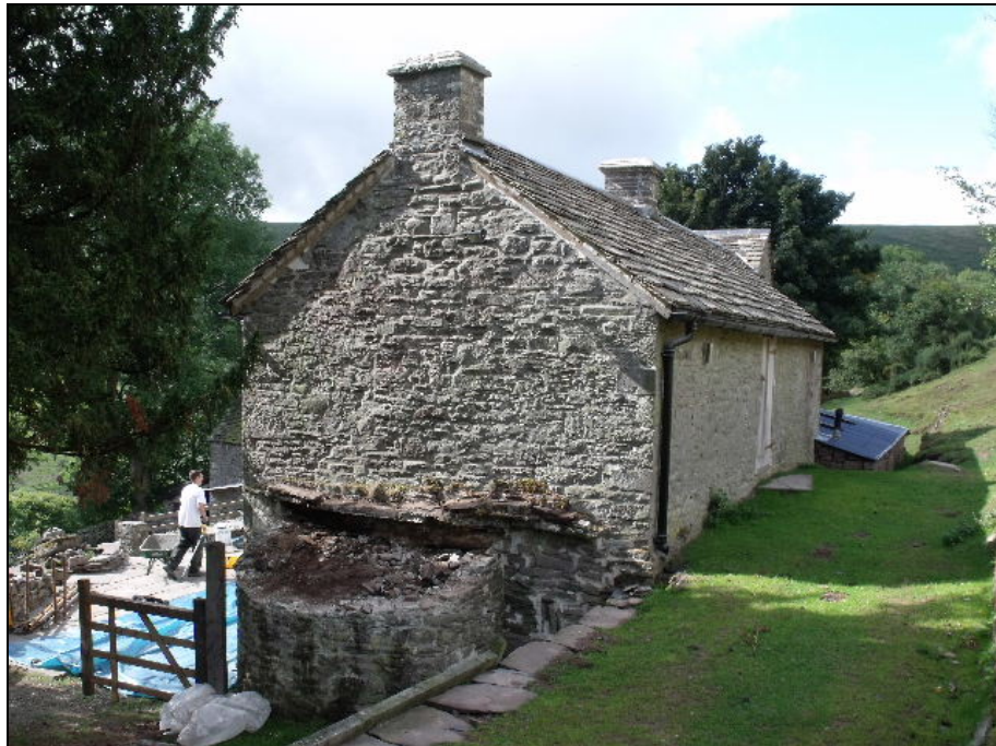
Fig. 2 The oven before the removal of the infill
