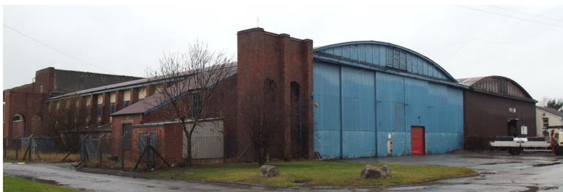
Plate 2: Listed General Service Shed (Belfast Truss Hangar) at the former RAF Sealand. Photo CPAT 3391-0042
