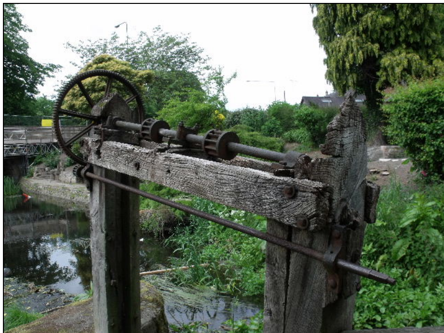
Fig. 5 The spillway sluice mechanism. Photo CPAT 3288-0014
