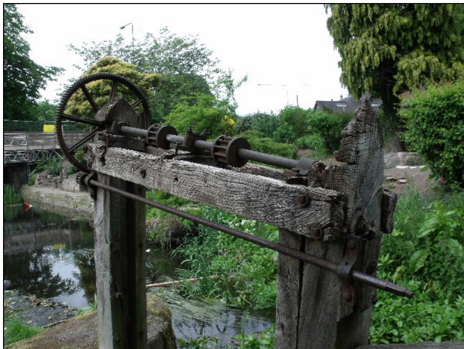
Fig. 5 The spillway sluice mechanism. Photo CPAT 3288-0014
