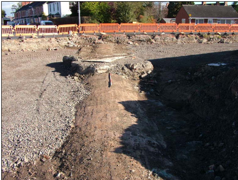
Plate 1: The top of the culvert carrying the Lledan Brook beneath Mill Lane (Photo CPAT 3199.0008)
