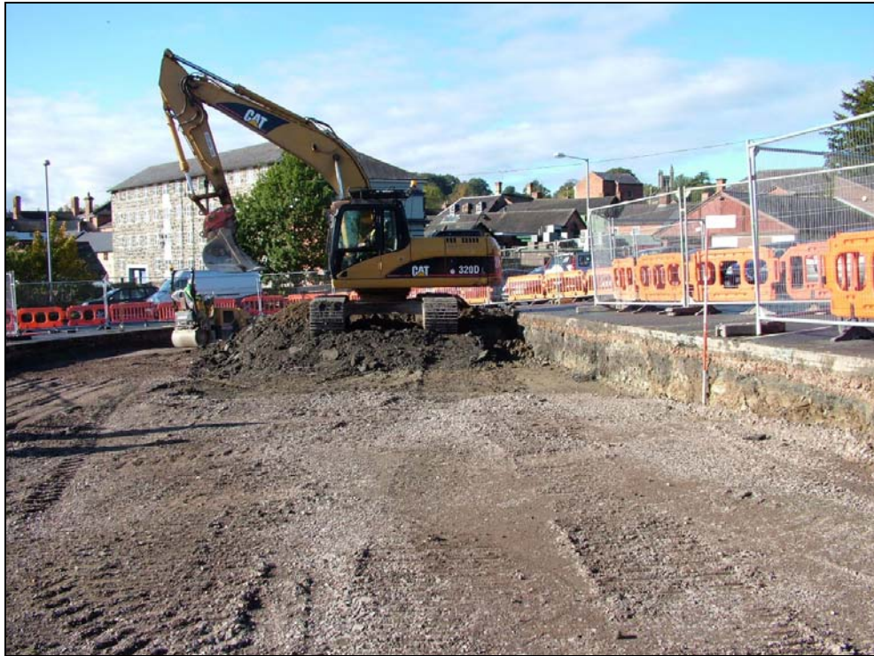
Plate 4: Machining of the new section of road across the car park (Photo CPAT 3199-0002)
