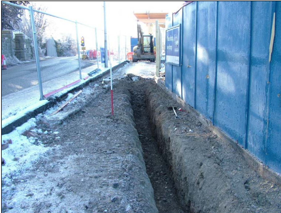
Plate 2: Excavation of the roadside drain opposite Domen Gastell motte and bailey castle (Photo CPAT 3199.0017)
