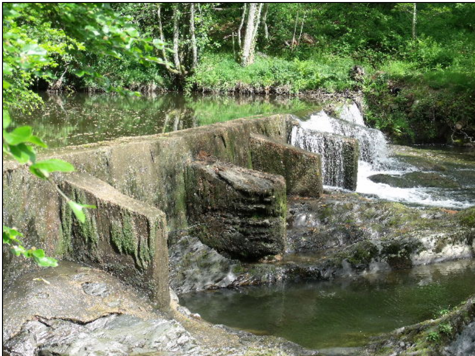
Fig. 5 The southern end of the weir showing the concrete section. Photo CPAT 3283.0015
