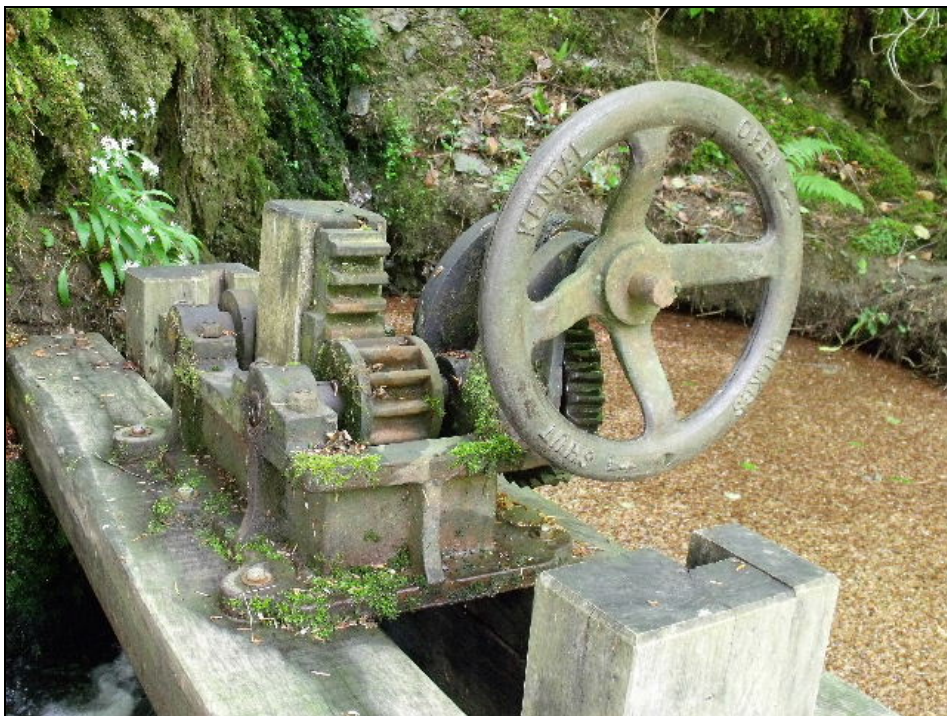
Fig. 7 The geared sluice controlling the feeder leat. Photo CPAT 3283.0012
