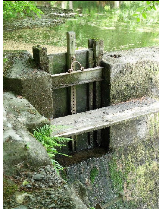
Fig. 6 The lifting sluice. Photo CPAT 3283.0014
