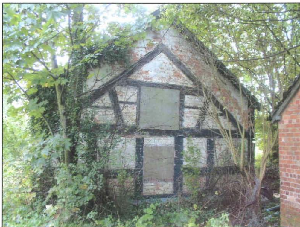
Plate 4 Western gable of Dolanog Cottages showing original roof line
