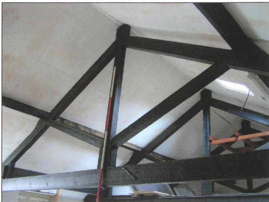
Plate 5 The exposed roof trusses above the upper floor (Photo CPAT 2575-052)
