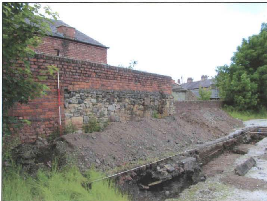
Plate 7 The stone-built section of wall to the rear of the bakery (Photo CPAT 2575-093)
