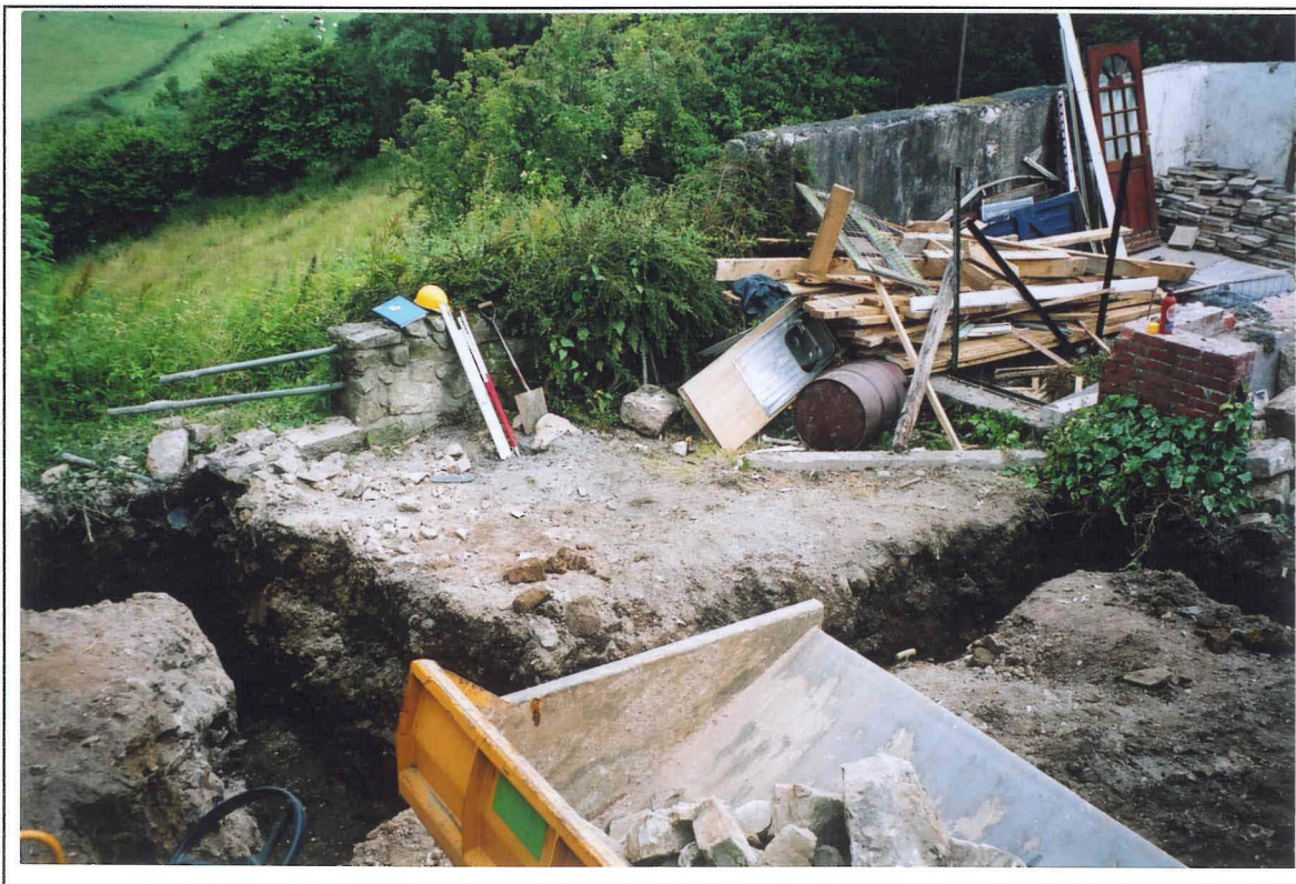
Plate 2. View from the south-east, showing footings excavated through 19th Century levelling deposits. The upstanding wall is along the projected line of Offa's Dyke. Photo CPAT 1714.04
