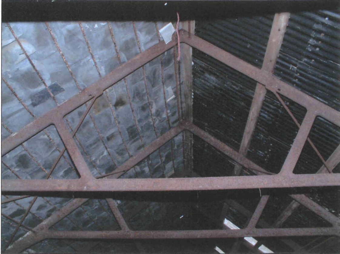
Plate 14 Barn 3 cast iron roof truss
