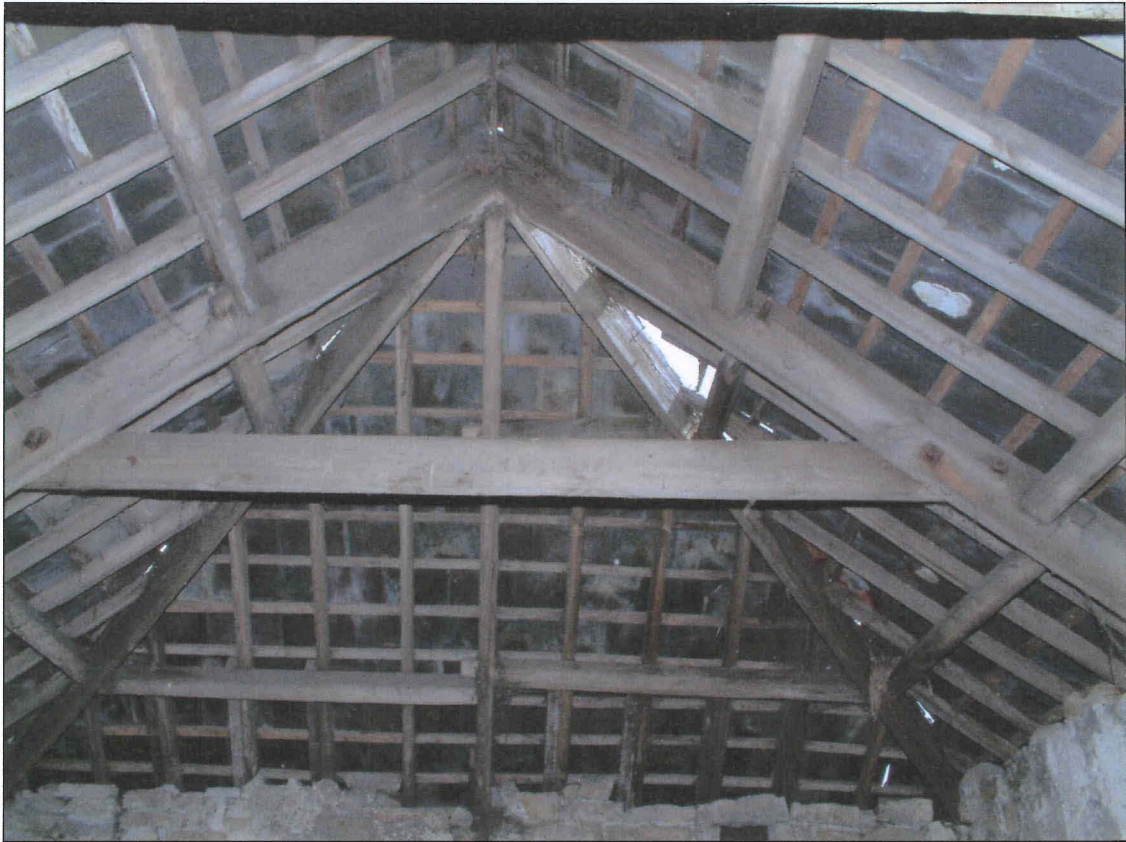
Plate 13 Barn 2 roof showing truss and hipped east end
