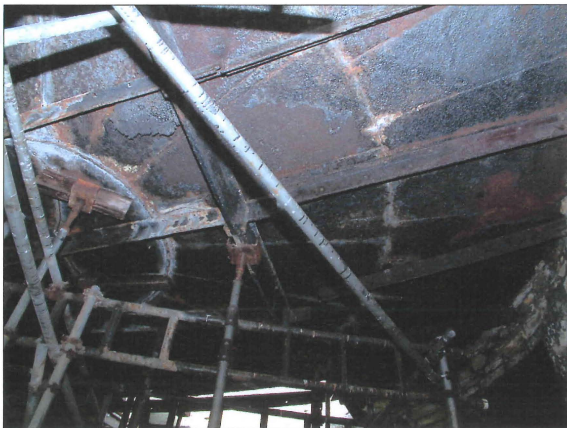
Plate 8 North-east tower, cast iron roof plates
