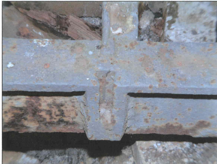
Plate 5 Detail of cast iron dove-tail joint
